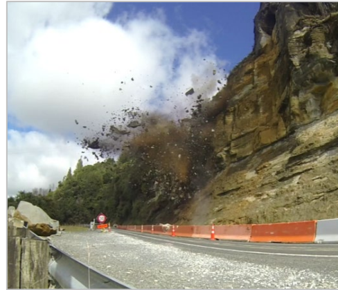
Blasting as part of rock stabilisation works at Mangaotaki Bluffs in May 2014
