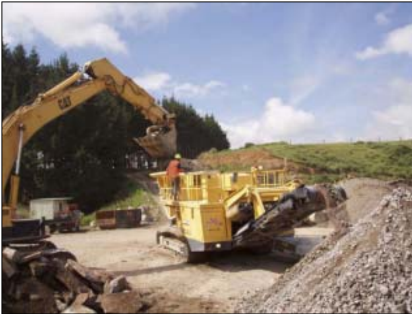
Photograph 5 Concrete being crushed at Jones Quarry. Photo credit: Nelle Rose
