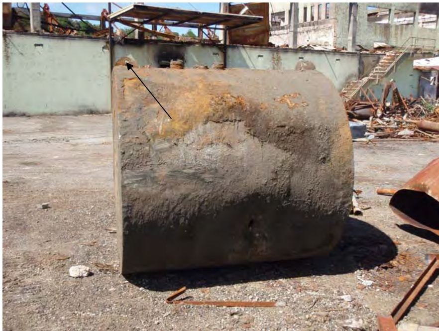
Photograph 2: Tank 1, 5000 L Diesel tank
