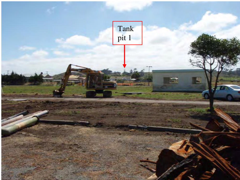
Photograph 6: View north towards site entrance and Tank Pit 1
