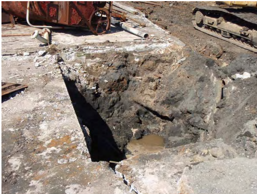
Photograph 4: Tank pit 2. Groundwater can be seen in base of tank pit.
