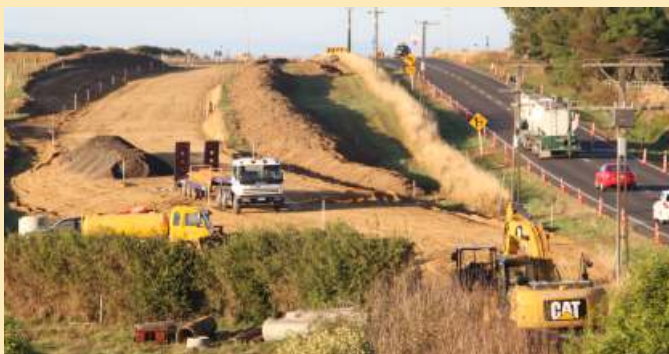
Work has started on the SH3 Normanby project.
