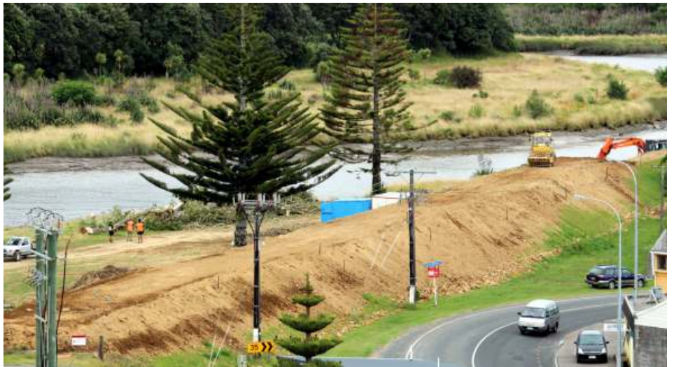
Contractors raise the stopbanks upstream of the Town Bridge.
