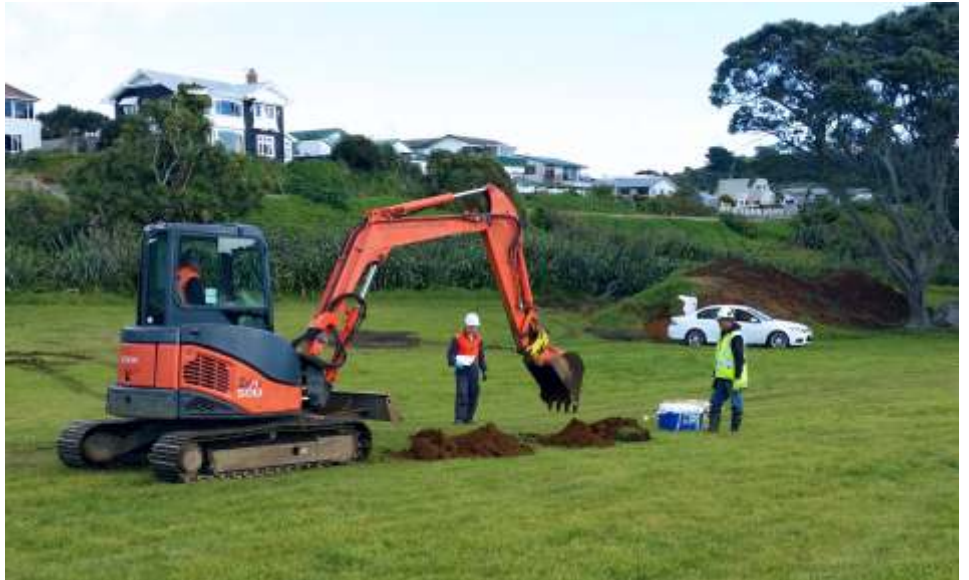
The Bayly Road site investigation included soil and groundwater sampling.
