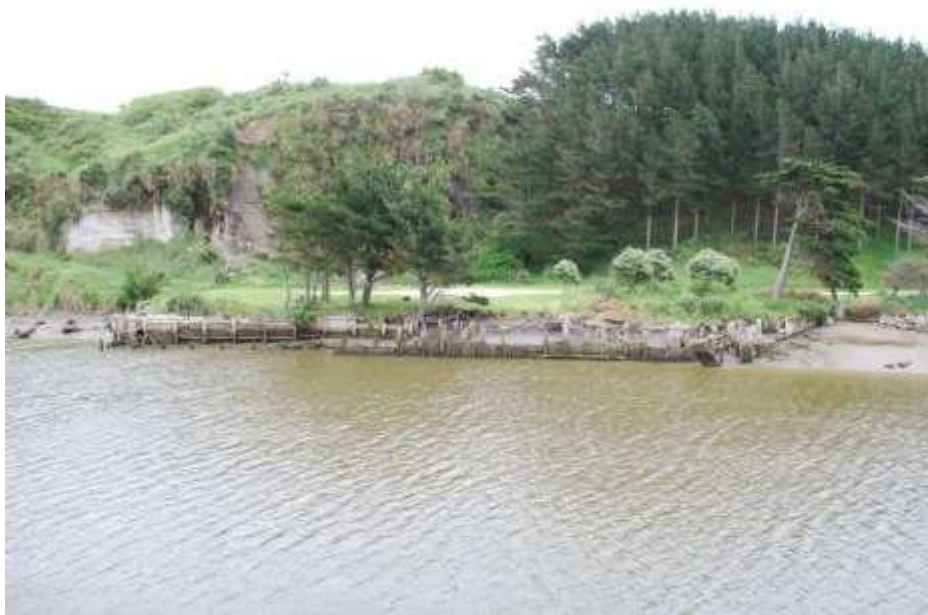
Figure 6: Town wharf remains at Pātea. Photo Ange Lenz, 2010
