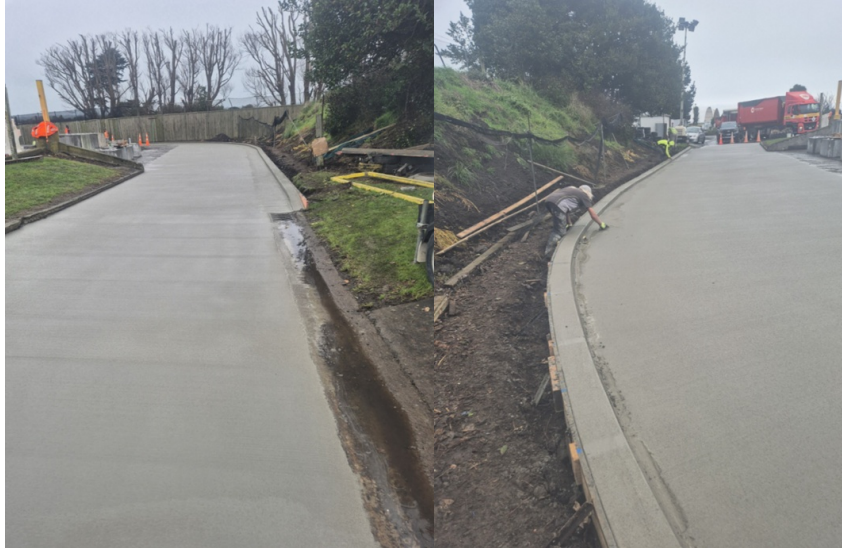
Figure 4 and Figure 5 Driveway and curb and channel improvements at the Hāwera Transfer Station
