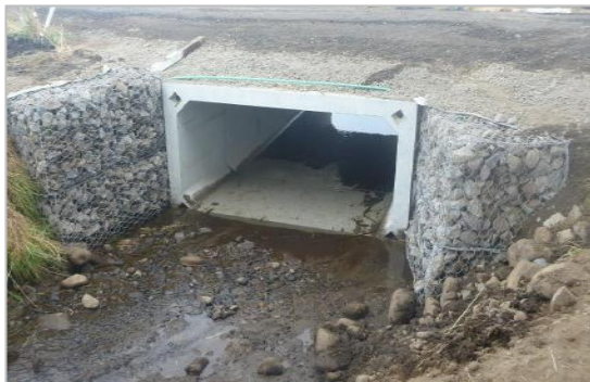
Bridge 117 – Wiremu Road
