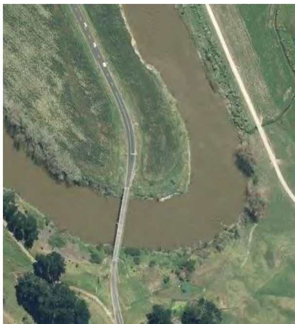
Figure 4-5: Site 3 - Limeworks Bridge Area before June 2015 Flood
