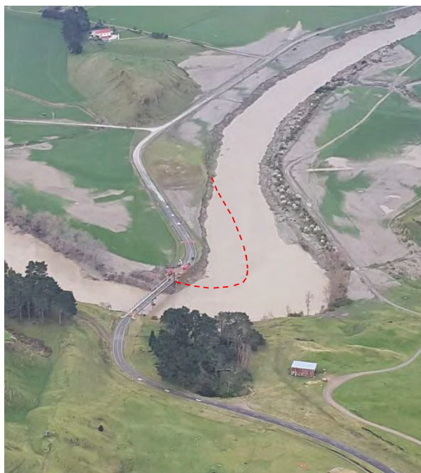
Figure 4-6: Site 3 - Limeworks Bridge after June 2015 Flood
