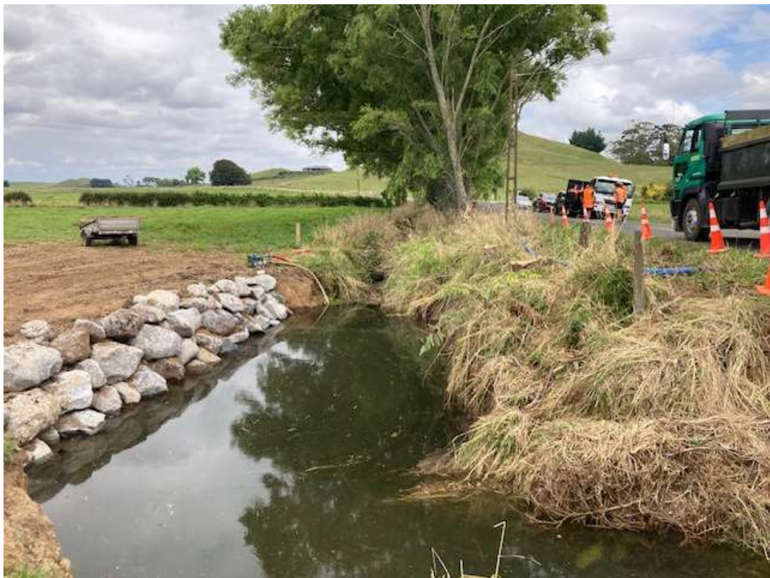
Figure 4: Rock armouring at the outlet of the new culvert.
