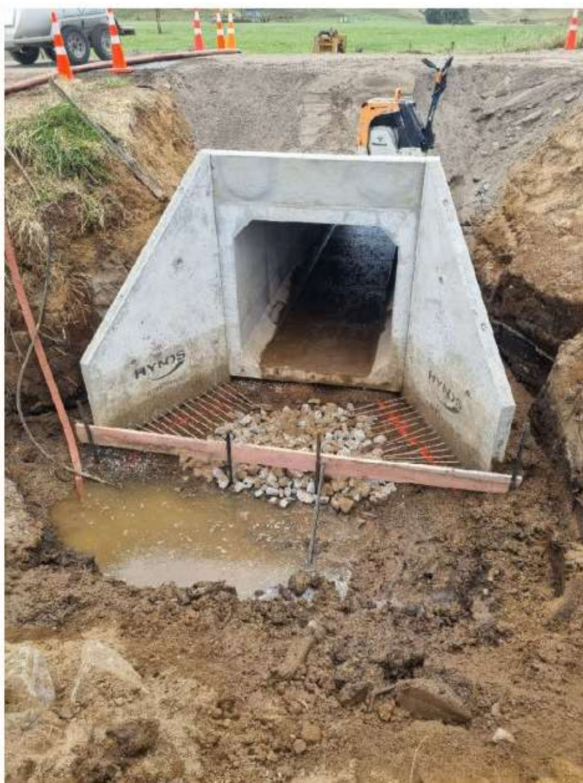
Figure 7: Box units in place and backfill over the culvert.
