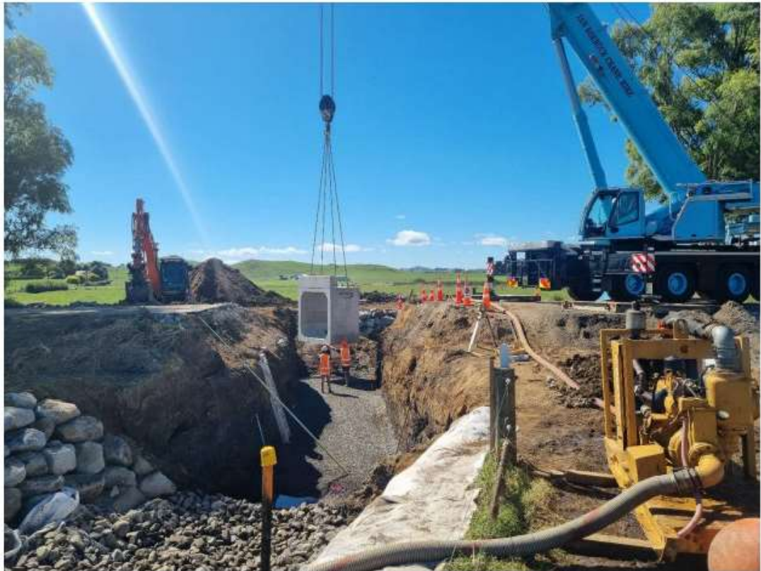
Figure 6: New pre-cast concrete box unit being lifted into place.
