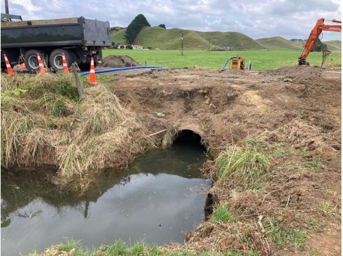
Figure 5: The inlet of the existing 1200mm diameter culvert.
