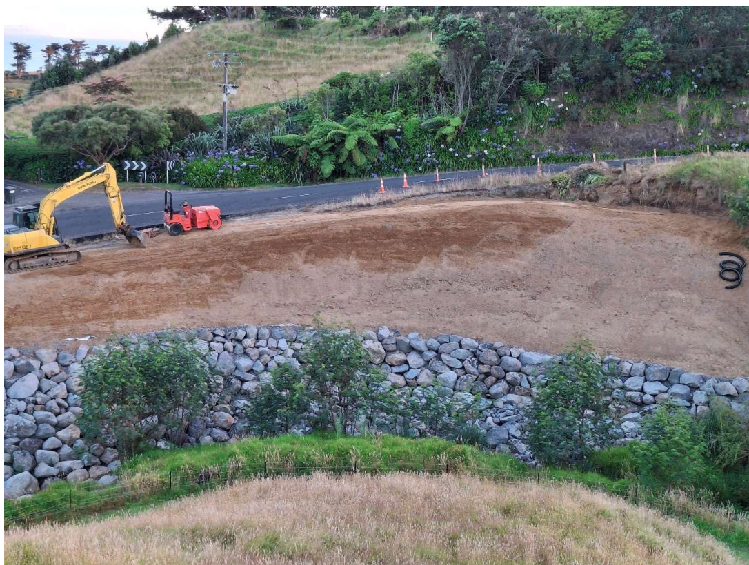
Picture – Surrey Hill Rd Underslip Repair
