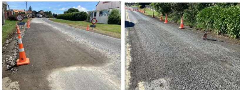
Figure 2: Pavement repairs on Cardiff Rd.
