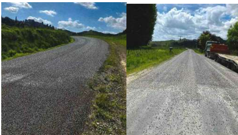
Figure 8: Two reseal sites on Mangaotuku Road undertaken in November 2024.
