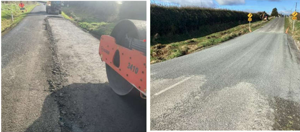
Figure 2: Seal widening of Salsbury Road
