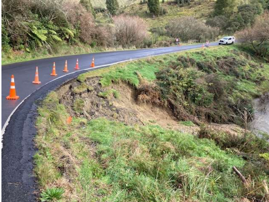
Figure 2: Mangaotuku Road under slip.
