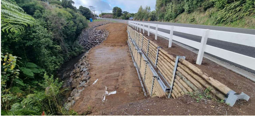
Figure 1: The steel piles being installed on Opunake Road.
