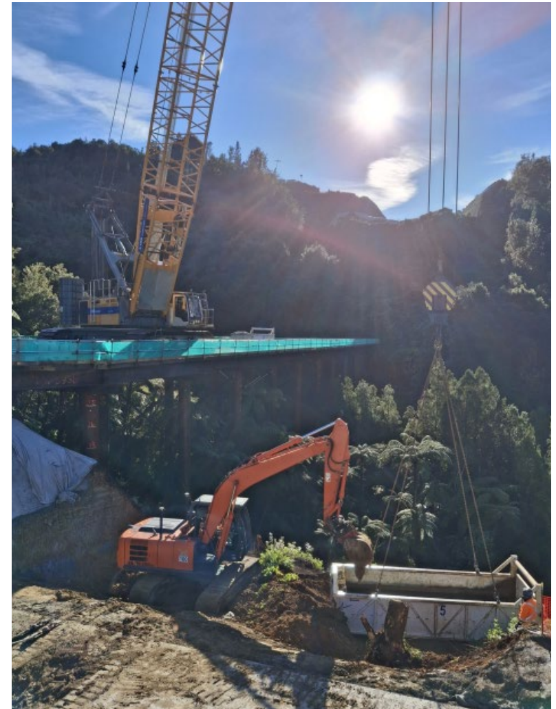
Temporary staging bridge is now complete.
