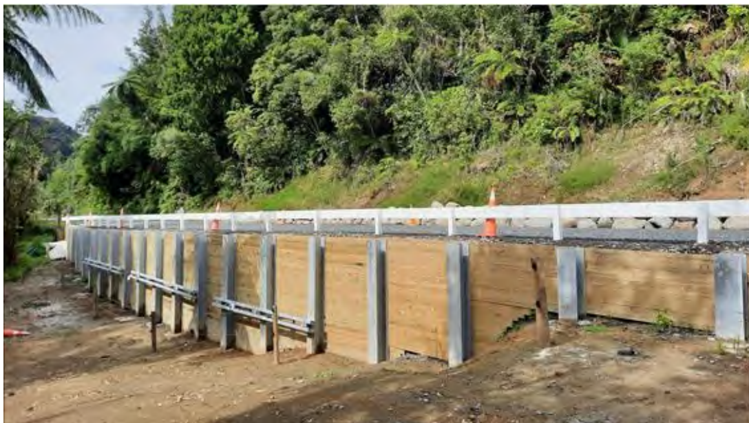
Picture - Okau Road retaining wall
