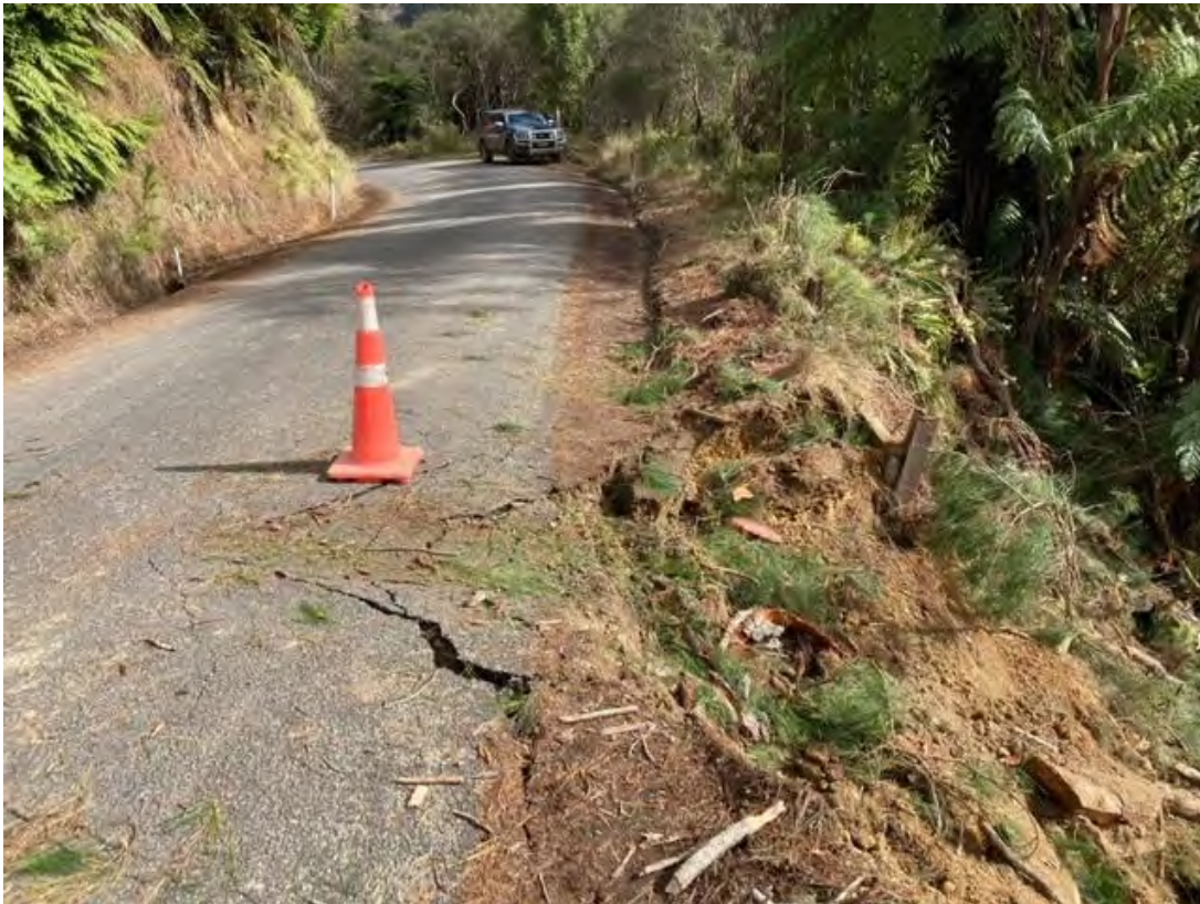
Figure 5: Damage to a retaining wall and road surface on Matau Road.
