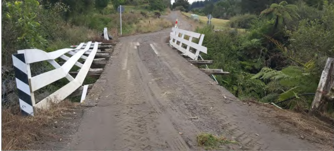
Figure 4: Damage to the bridge located at the end of Puniwhakau Rd.
