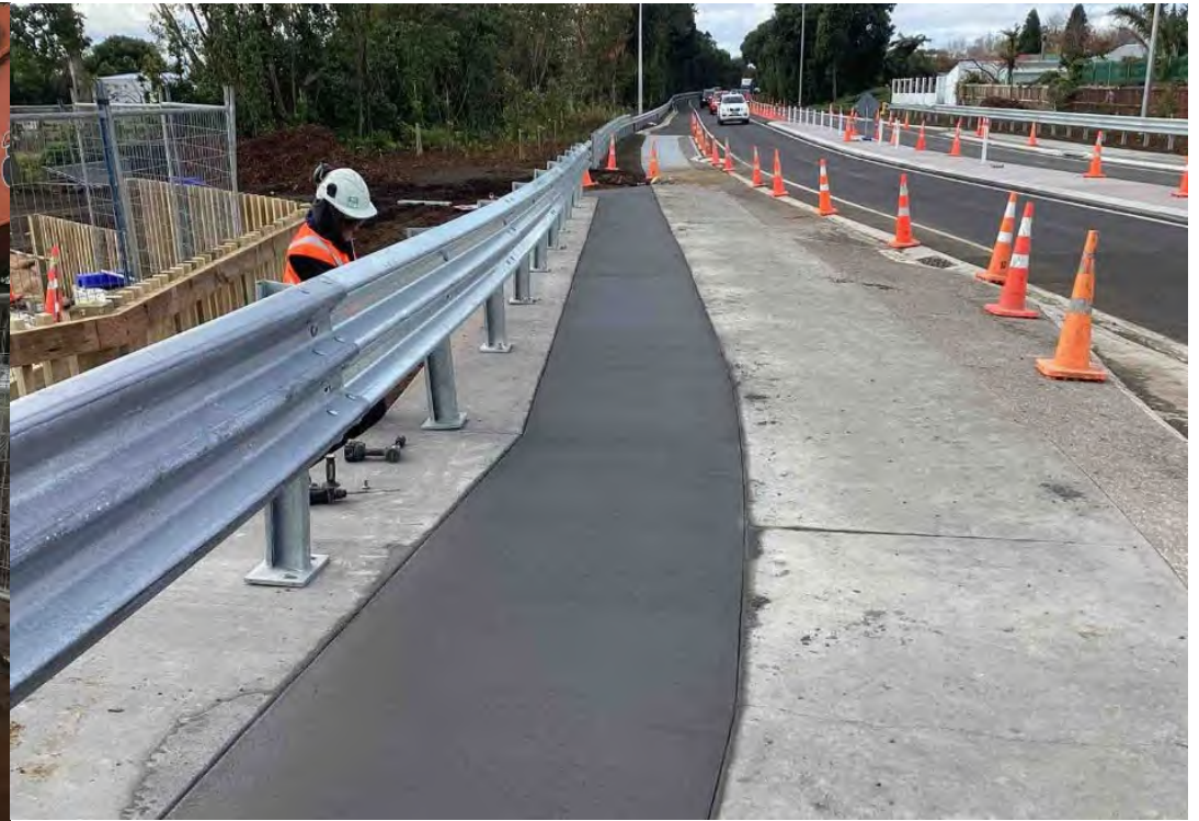
Image: Guardrail installation at Princess Street
