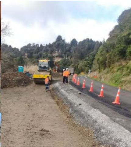
Work underway at Mangaotaki underslip
