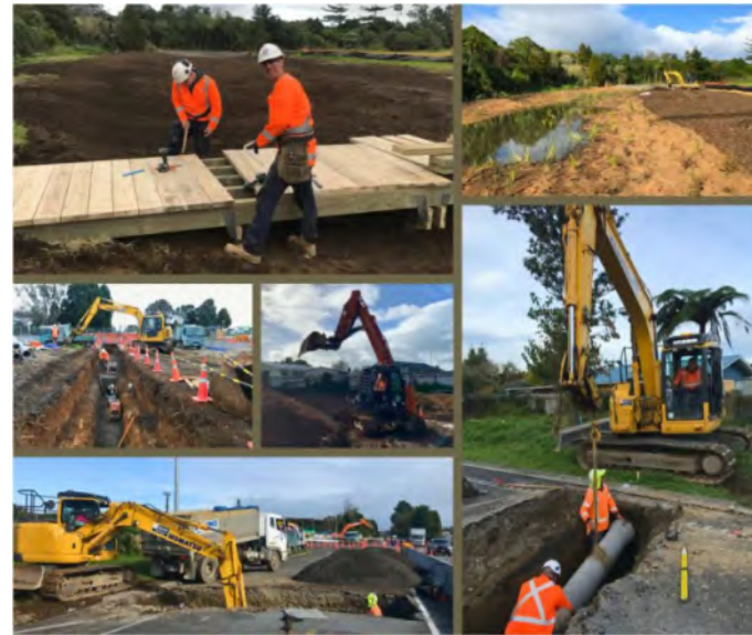
Work underway at Princess Street intersection and Manukorihi swale
