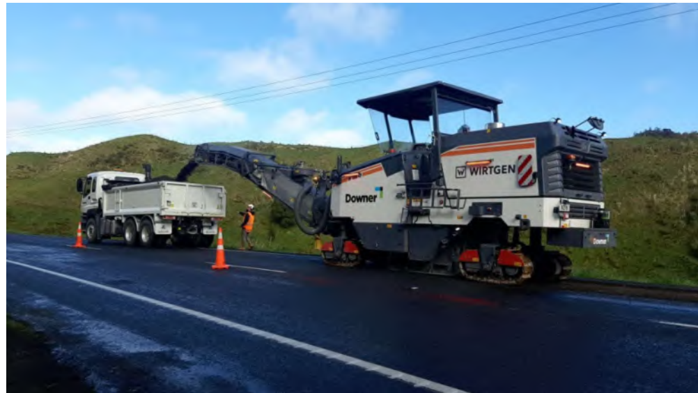
Milling machine in action on SH3 near Uruti
