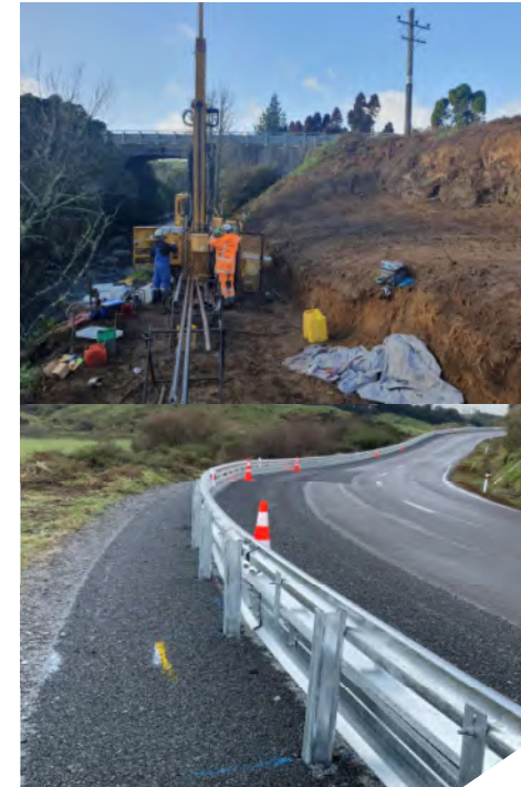
Top image: Proof drilling at Kahouri Stream Bridge Bottom image: New guardrail with motorcycle protection installed on SH43
