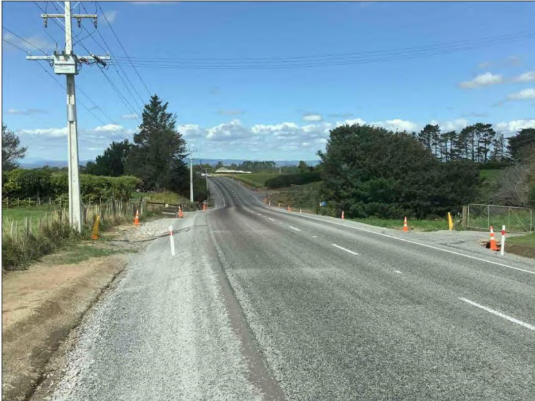
Figure 1 – Monmouth Road Rehab following the sealing of the road.
