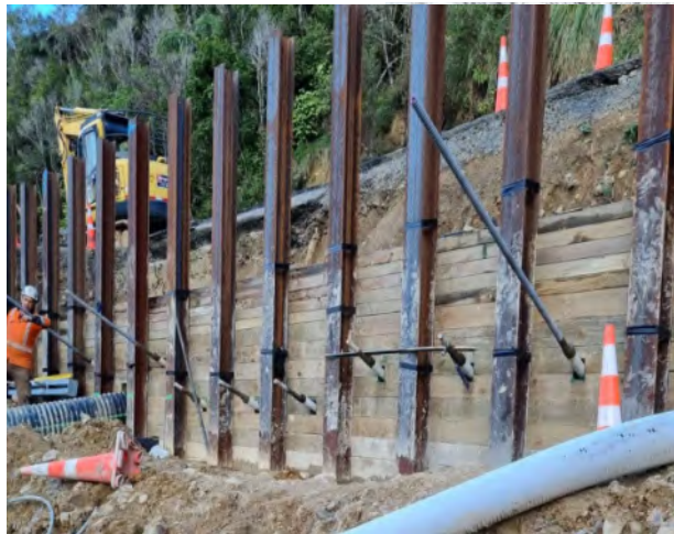
Retaining wall construction at Awakau Road
