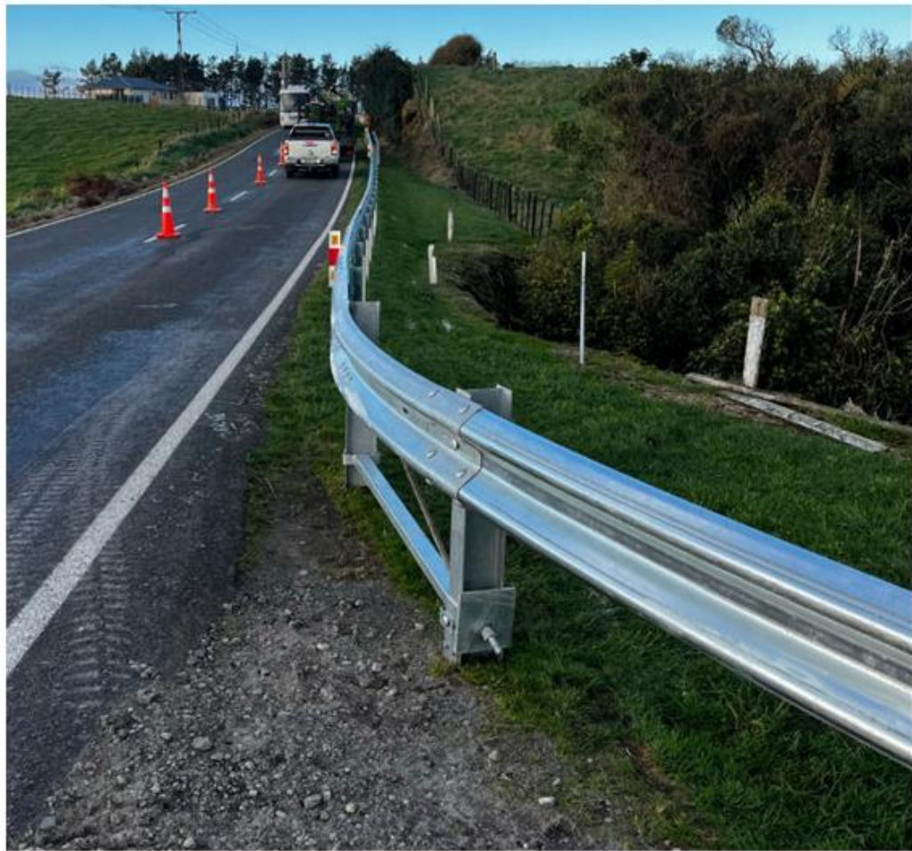
Figure 7 – Roadside Barrier at 343 Opunake Road.
