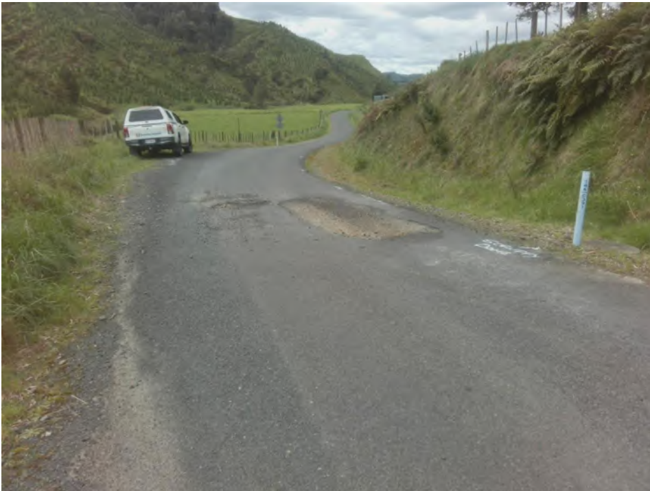
Figure 2 – Pavement Failure on Matau Rd.
