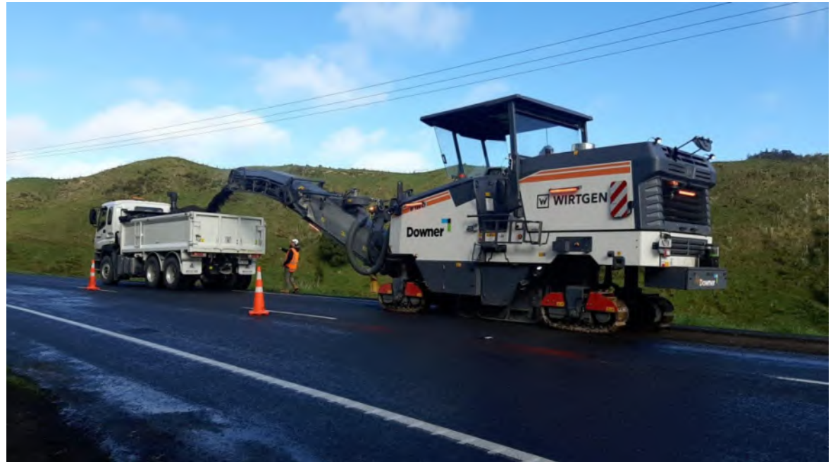
Milling machine in action on SH3 near Uruti
