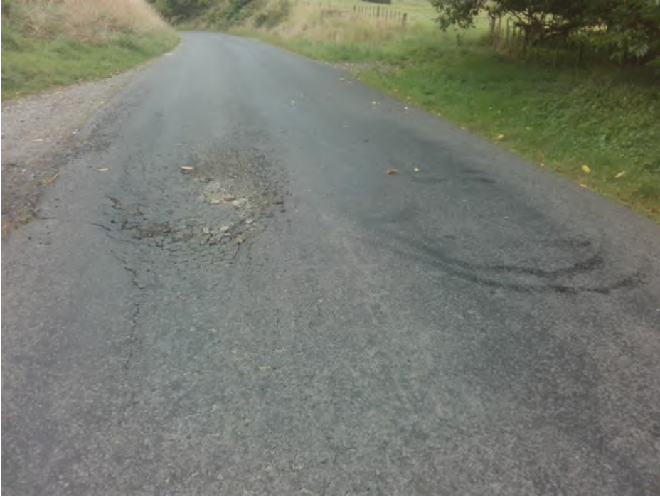
Figure 1 – Pavement Failure on Brewer Rd. This is just one of many similar faults that require repairs.
