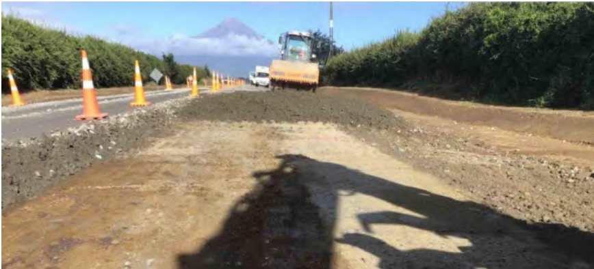
Figure 3 – Monmouth Rd – Pavement digout
