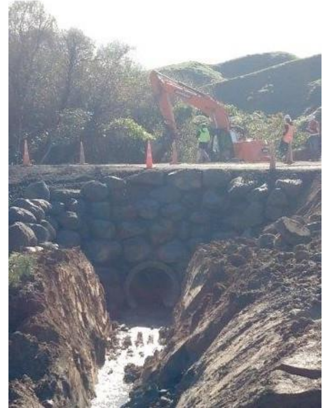
SH3 Awakino culvert collapse
