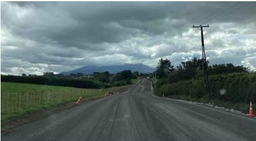
Figure 4 – Granular Overlay
