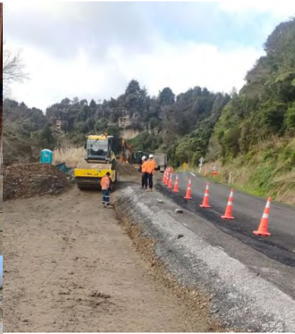
Work underway at Mangaotaki underslip
