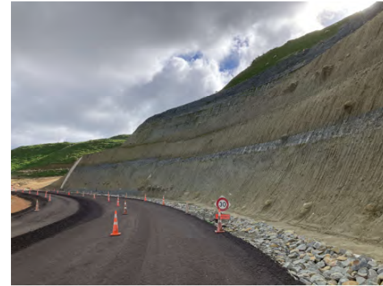
Auraki Stream road retreat project – new section of road
