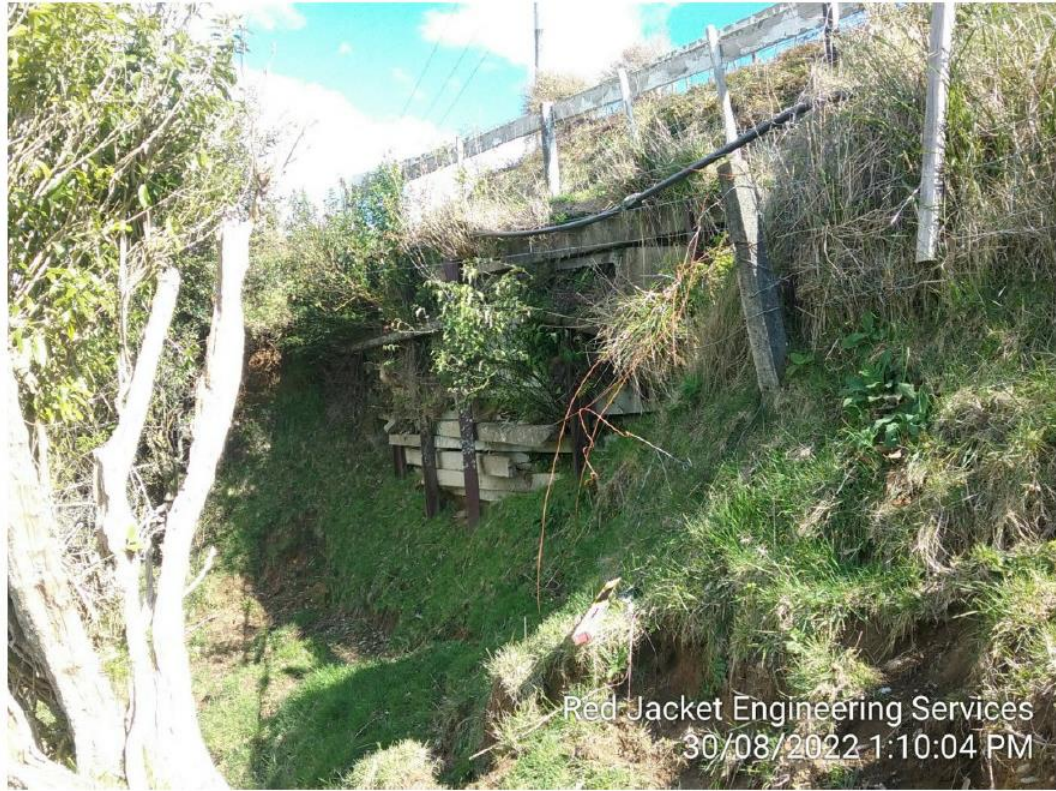
Figure 2 – Croydon Rd retaining wall to be replaced.
