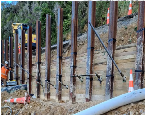
Retaining wall construction at Awakau Road
