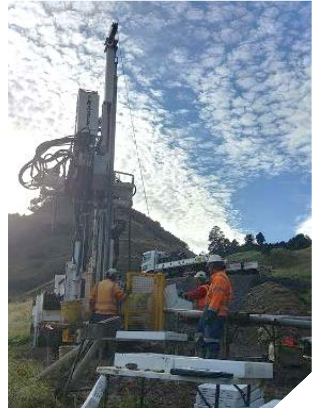
The crew at Te Oreore site drilling boreholes and installing groundwater monitoring devices, deep within the landslide area
