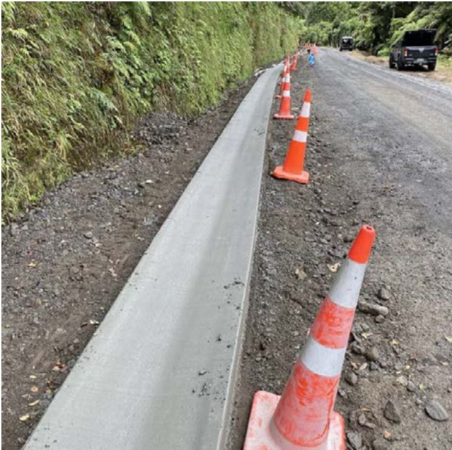
Concrete dish channel
