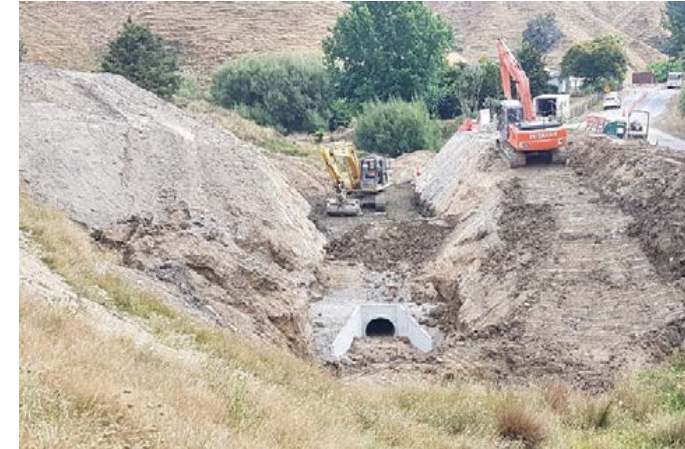
Image above shows Tahora Saddle work site
