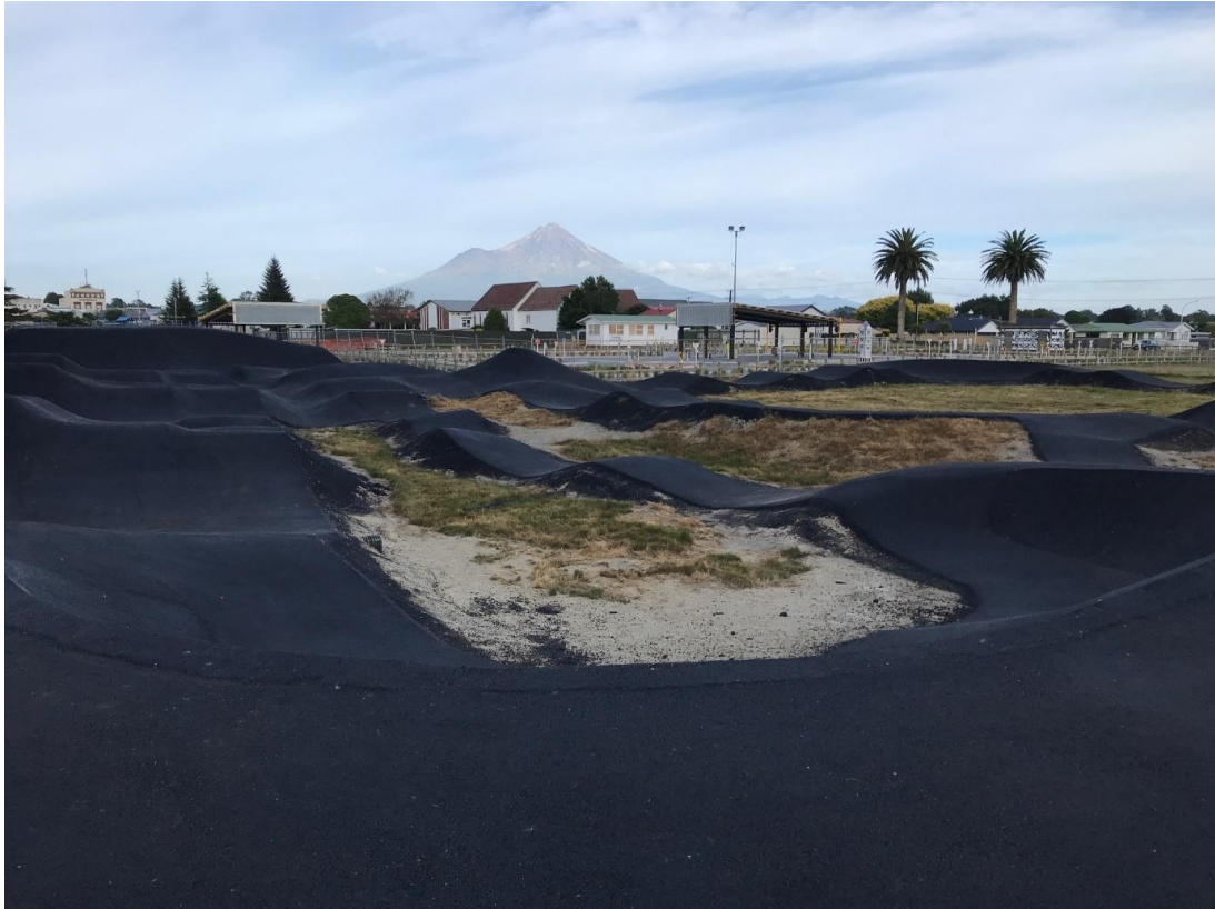
Figure 8 - The pump track with the asphalt surfacing.
