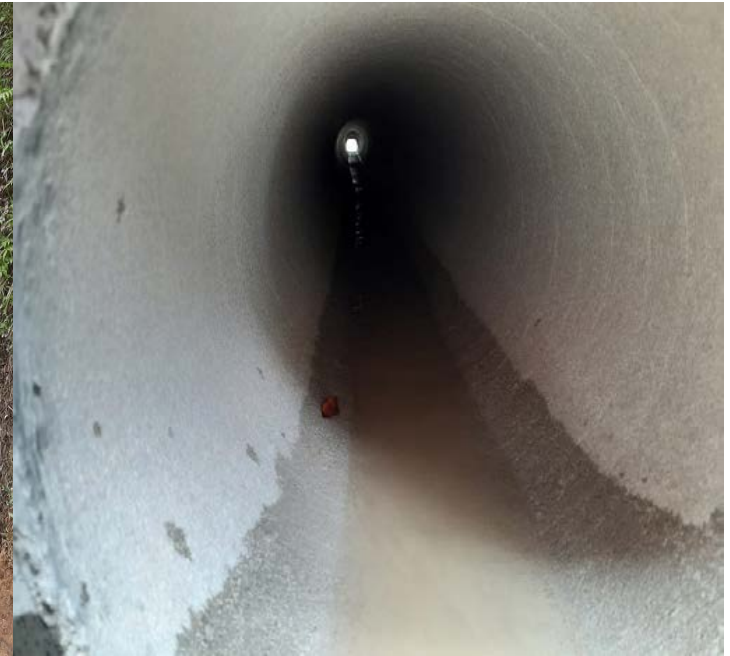
Newly installed culvert pipe
