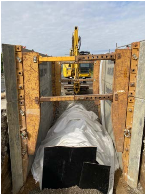
The new stormwater pipe installed
