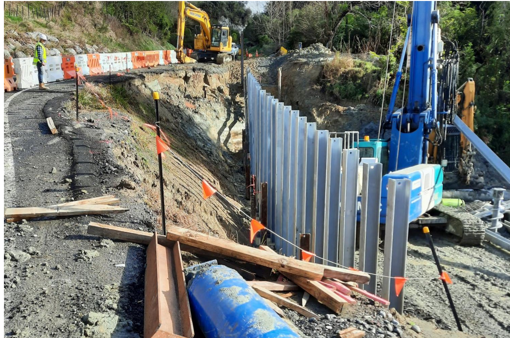
Retaining wall piles installed at site
