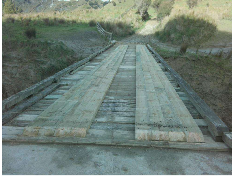
Figure 1: New timber running boards on the Matau North Road Bridge No.5
