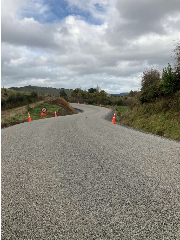
Figure 3 – Work in progress at Baldock's Corner on Mangaotuku Rd.
