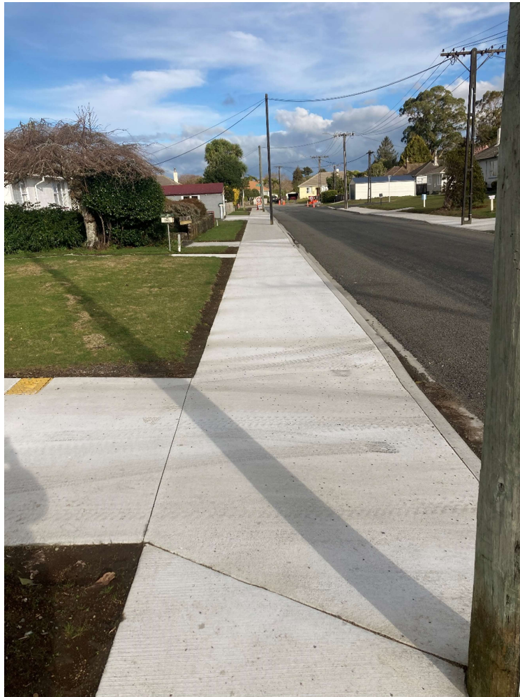
Figure 2 – Footpath replacement on Essex Street.
