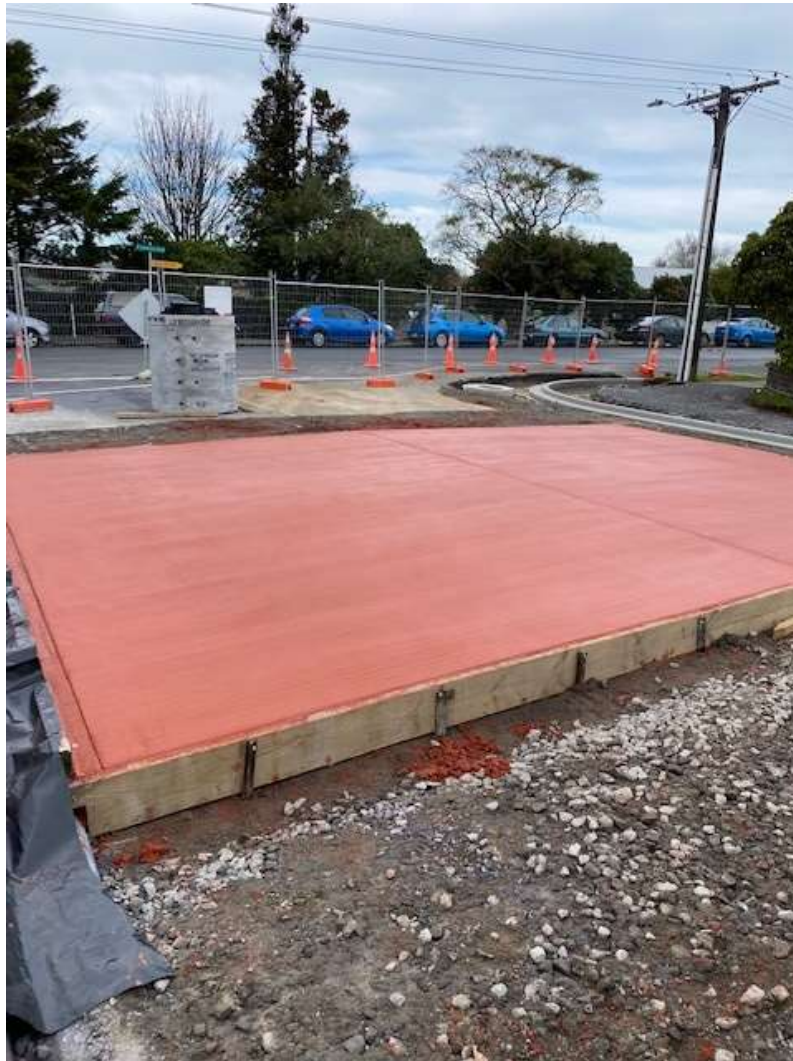
Figure 13 – Newly poured red concrete raised platform at Fenton Street/Swansea Rd intersection.
