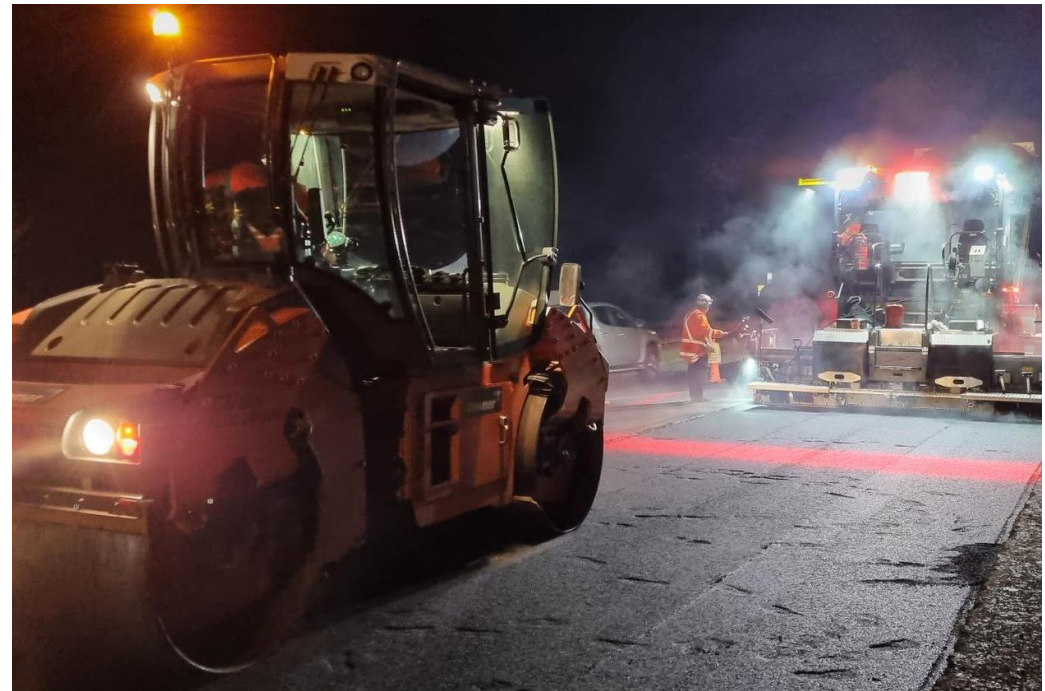
Asphalting at Eltham this season
