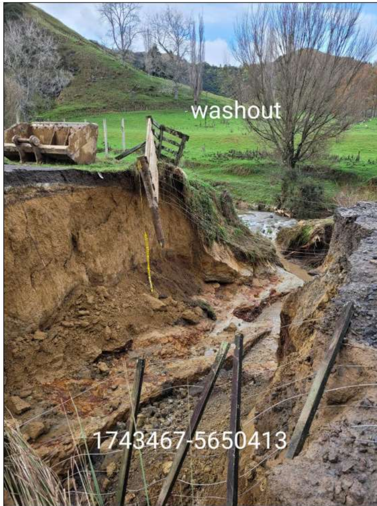
Figure 7 – The washout on Upper Mangaehu Rd just east of Murcott Road.
