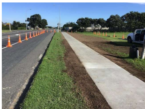
Tasman Street, Opunake new footpath
