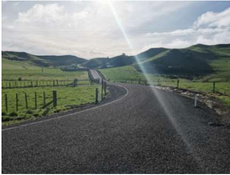
Hu Road, Eltham Pavement Rehabilitation
