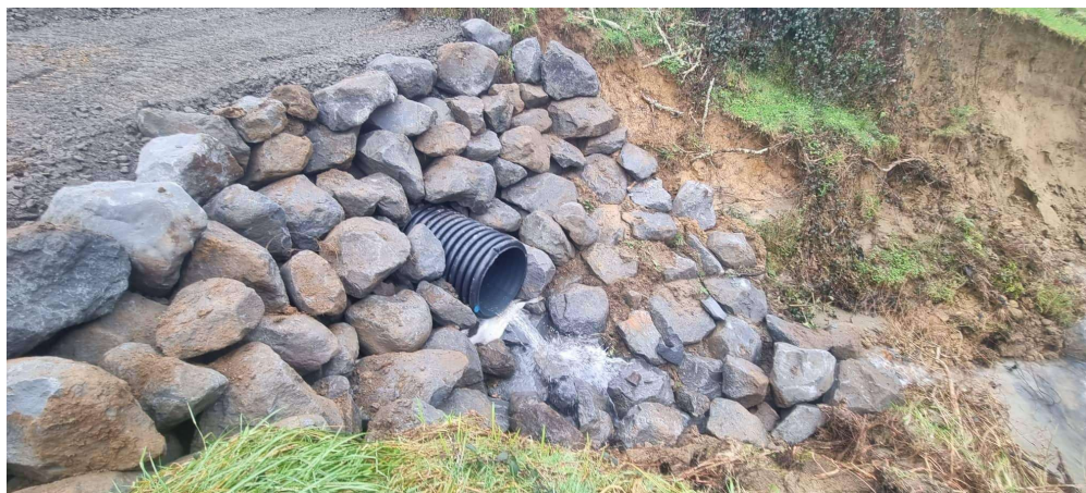
Figure 7 – The washout on Upper Mangaehu Rd just east of Murcott Road.
