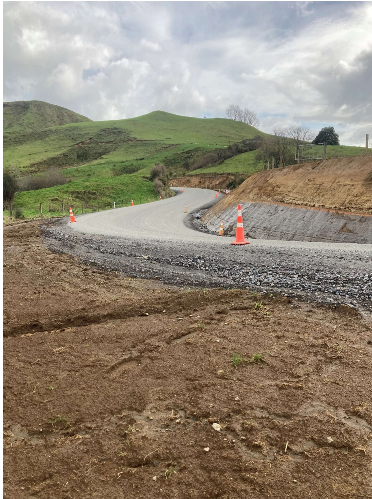
Figure 4 – Mangaotuku Road - note the bank trim on the right hand side.
