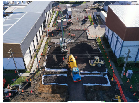
Tauhuri Street pavement works
