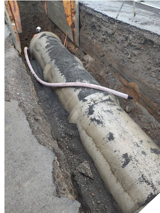
Stormwater pipe installed
