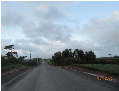
Bayly Road Pavement Rehabilitation
