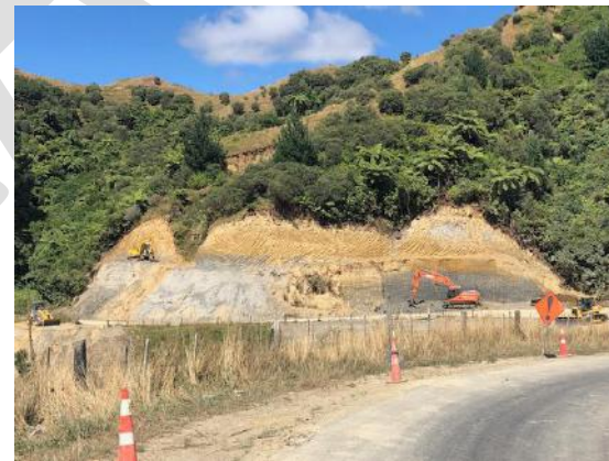
Mangaotuku Road Realignment
