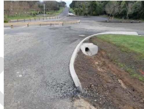
Shifting the entrance to the Hawera Cemetery due to existing intersection having a very poor sight visibility.
