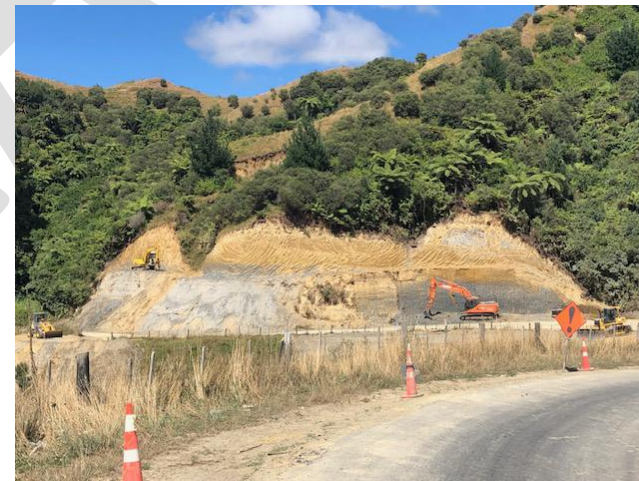
Mangaotuku Road Realignment
