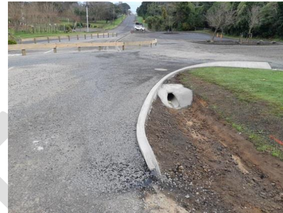
Shifting the entrance to the Hawera Cemetery due to existing intersection having a very poor sight visibility.
