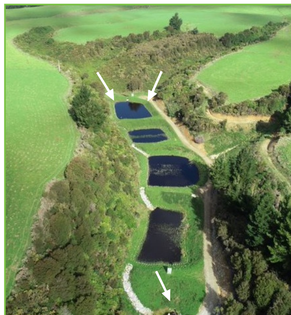
Stepped series of wetland cells constructed in a natural gully viewed from the inlet (left) and outlet (right) ends. Wetland plantings are still establishing.
