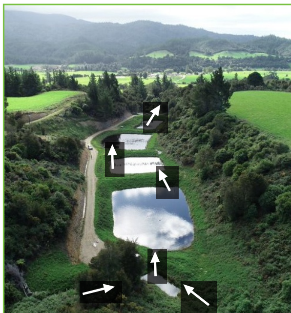
Stepped series of wetland cells constructed in a natural gully viewed from the inlet (left) and outlet (right) ends. Wetland plantings are still establishing.
