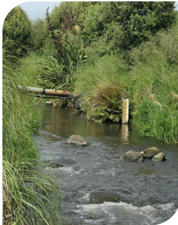
Hydrology gauge and water intake pipe, Waiokura Stream
