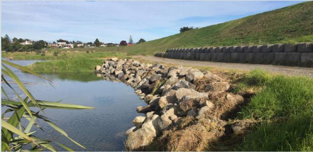
Image: Waitara River stopbank and erosion control.
