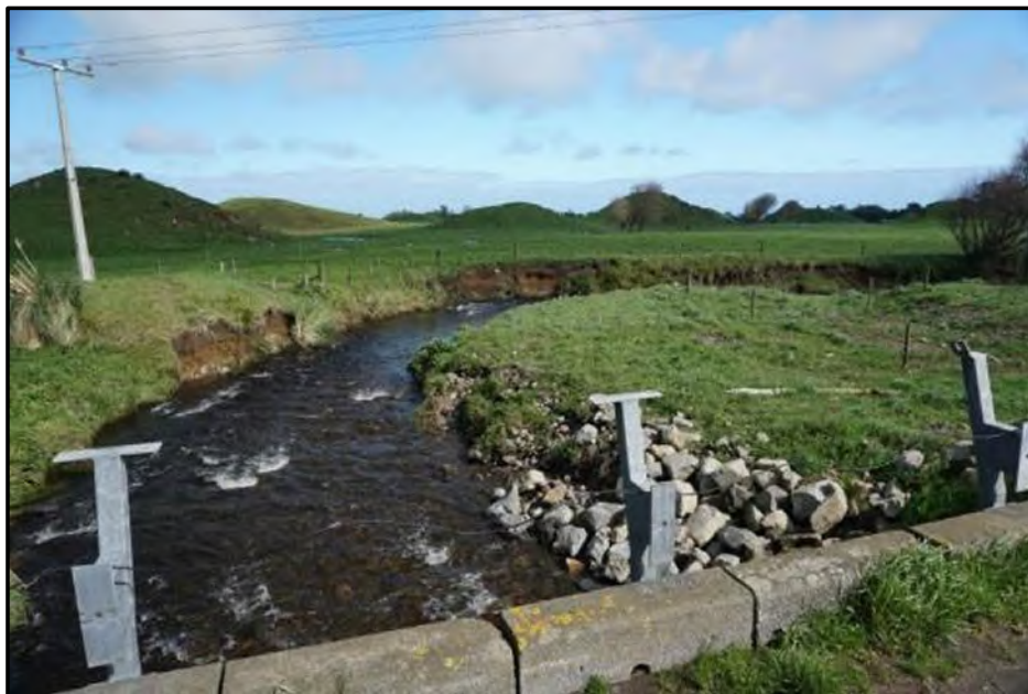
Figure 56. Example of hard structure (bridge) with localised erosion.
