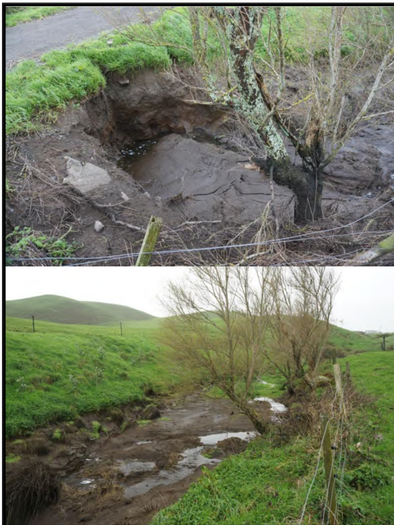
Figure 54. Example of a blocked culvert creating localised sedimentation.
