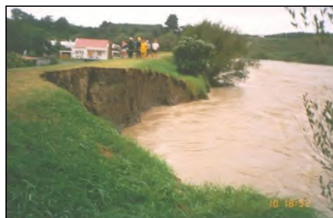
Figure 3: Waitara River bank collapse – 1990
