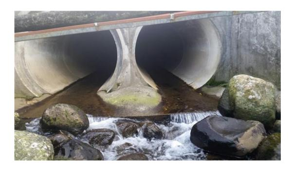
The above photo is an example of a non-compliant culvert, inspected in 2015. This culvert has now been retrofitted with staggered baffles to slow flow through the culvert, and the streambed has been built up downstream of the culvert, to remediate the perched apron.
