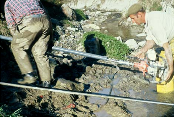
Figure 6. The drilling of a horizontal bore.
