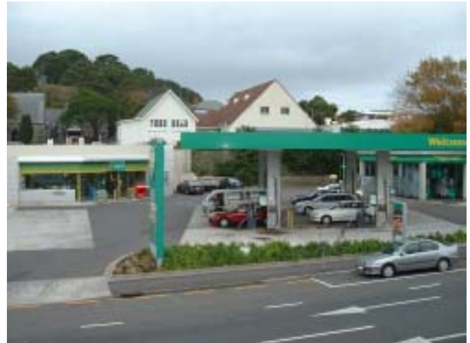
Photo 1: A service station has many sources of potential pollution. Follow the best management practices outlined in this information sheet
