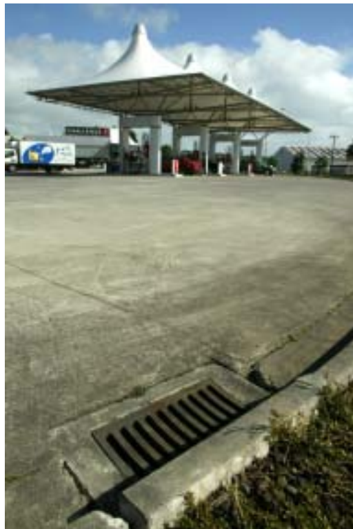
Photo 2: Stormwater runoff from the forecourt area flows to an interceptor system to remove potential contamination.
