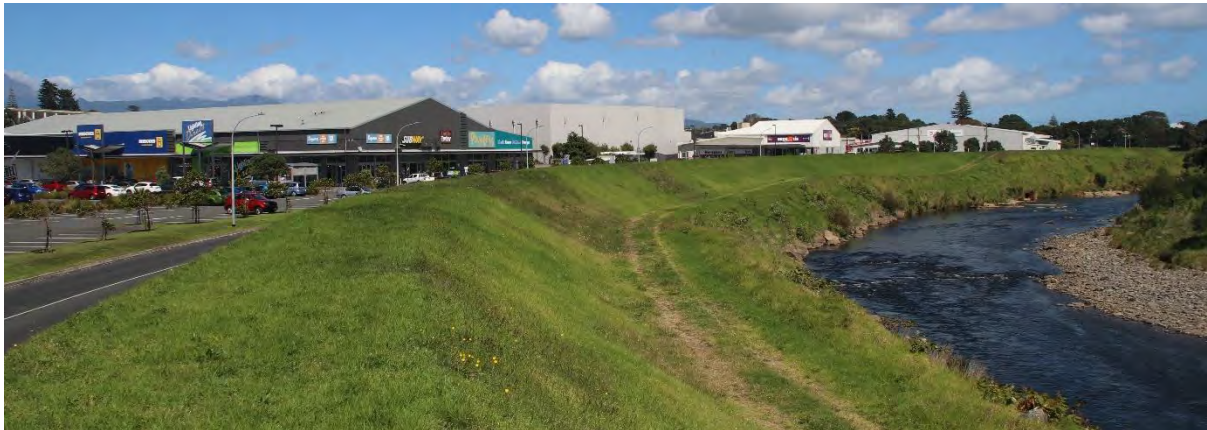
Part of Lower Waiwhakaiho River's current flood defences.
