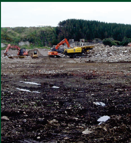
Removal of above-ground structures.
