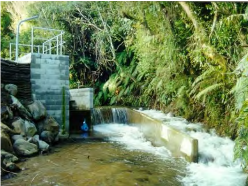
Photo 2 Downstream weir and fish pass in the Mangatoki Stream for the Inaha WTP
