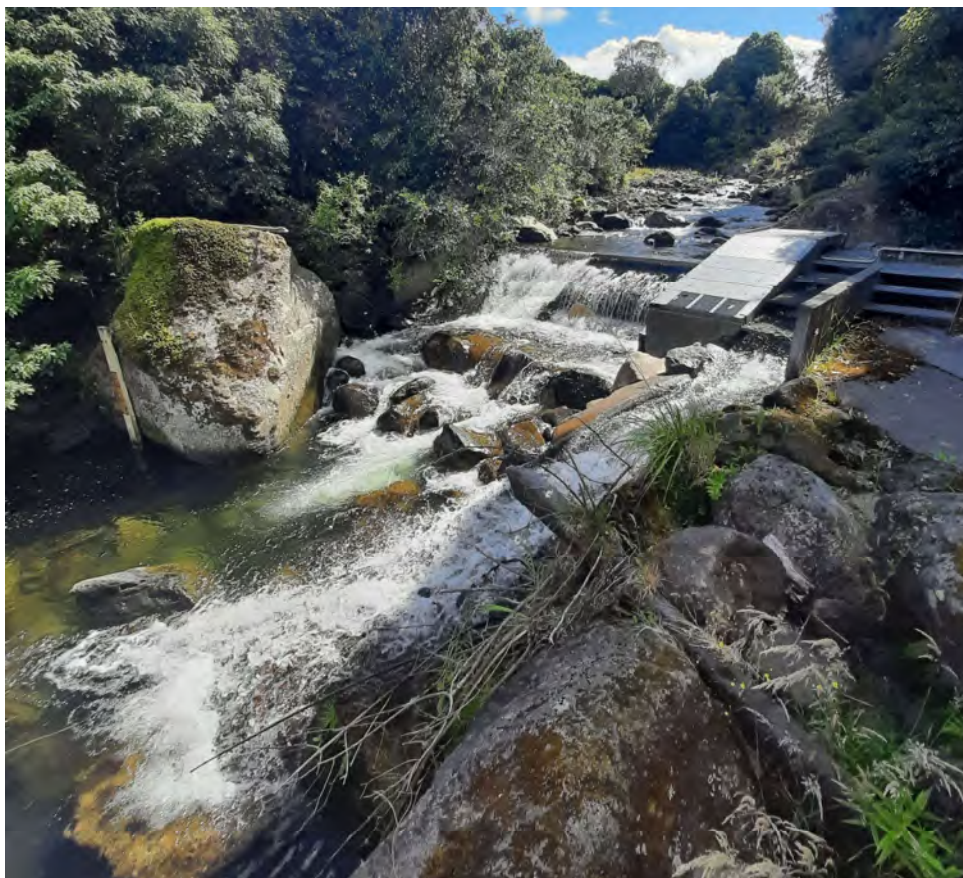
Photo 3 Downstream side of the STDC weir and fish pass in the Otakeho Stream for the Waimate West WTP
