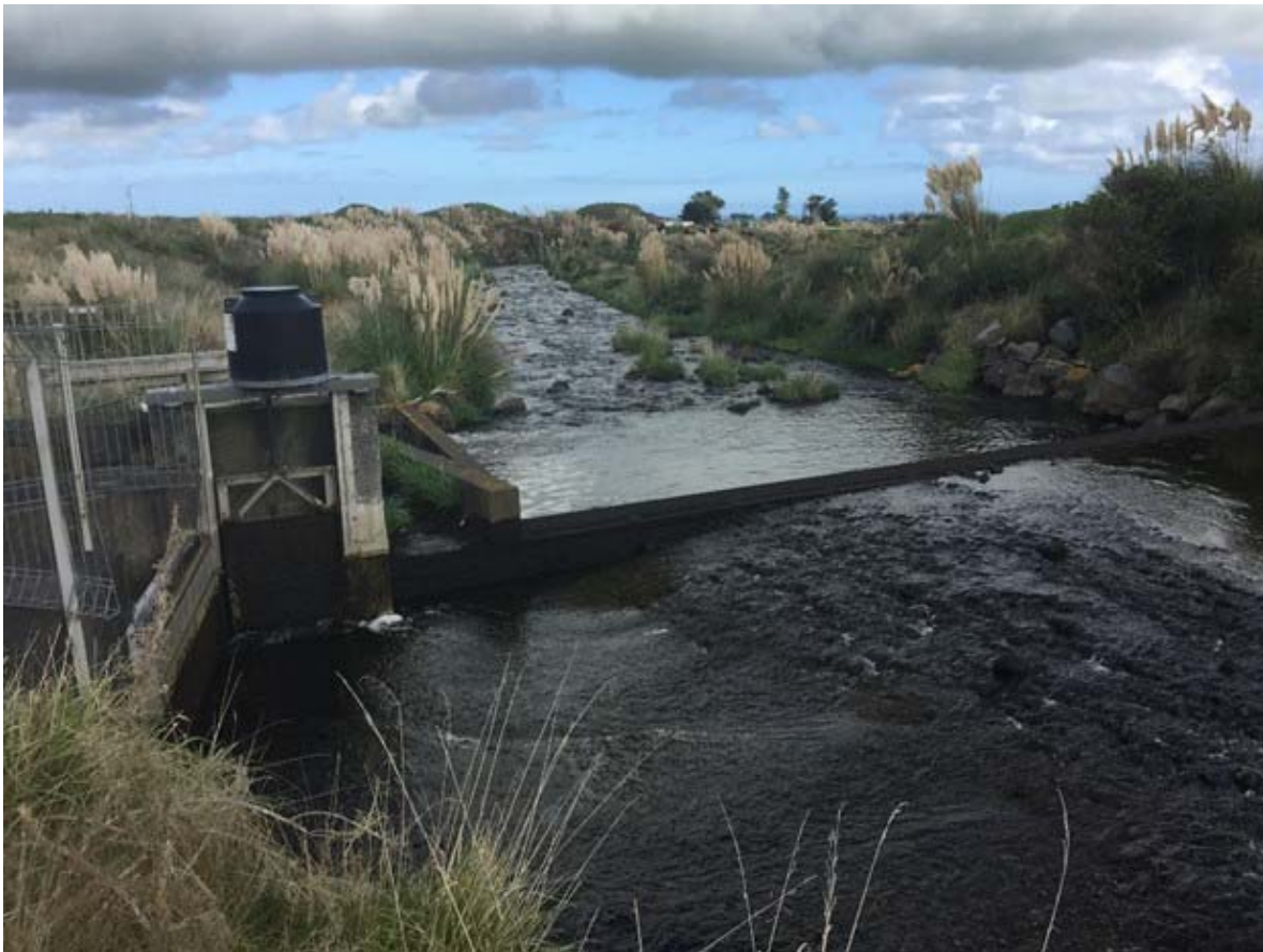
Photo 1 Water no longer flowing over the Oaonui water supply weir during a sluice
