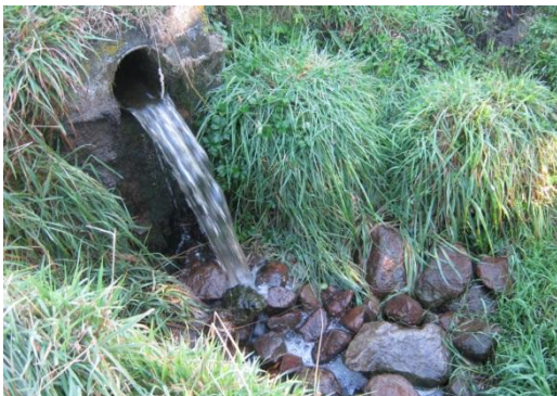
Photo 5 The small discharge channel from the oxidation ponds wetlands system prior to the Manaia Creek
