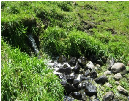
Photo 3 Additional rock rip-rap in the wetlands discharge channel, November 2013
