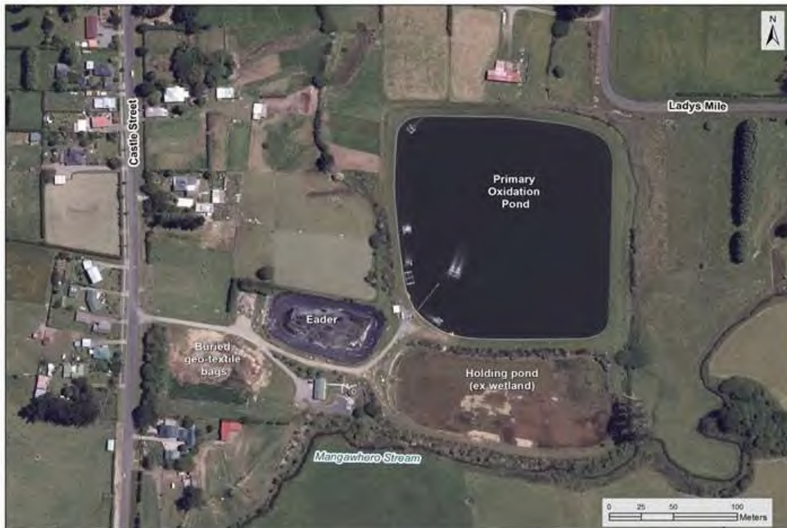
Figure 2 Aerial view of the Eltham WWTW
