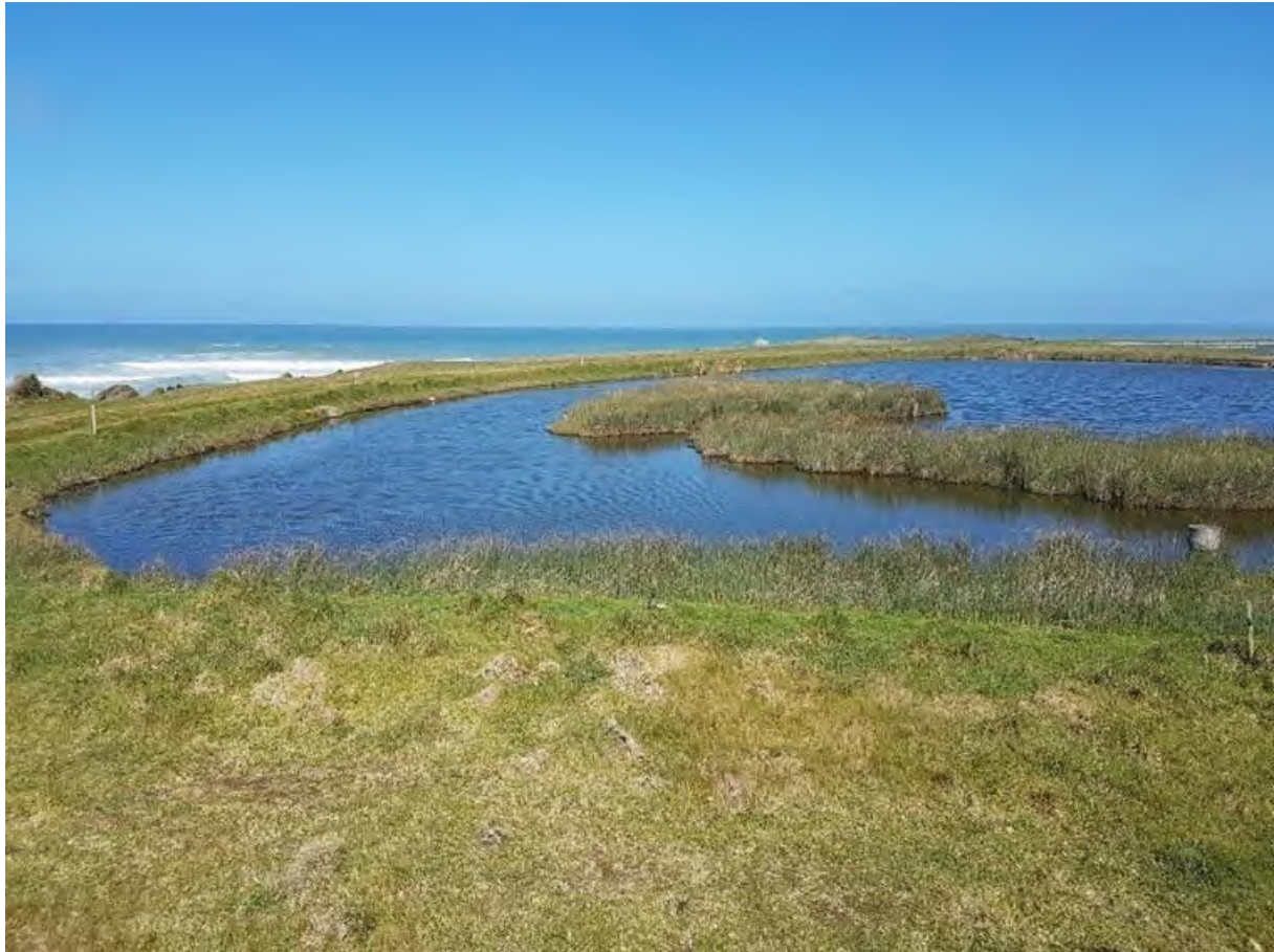
Photo 1 Opunake WWTP wetlands
