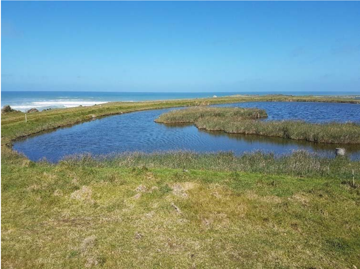
Photo 1 Ōpunake WWTP wetlands
