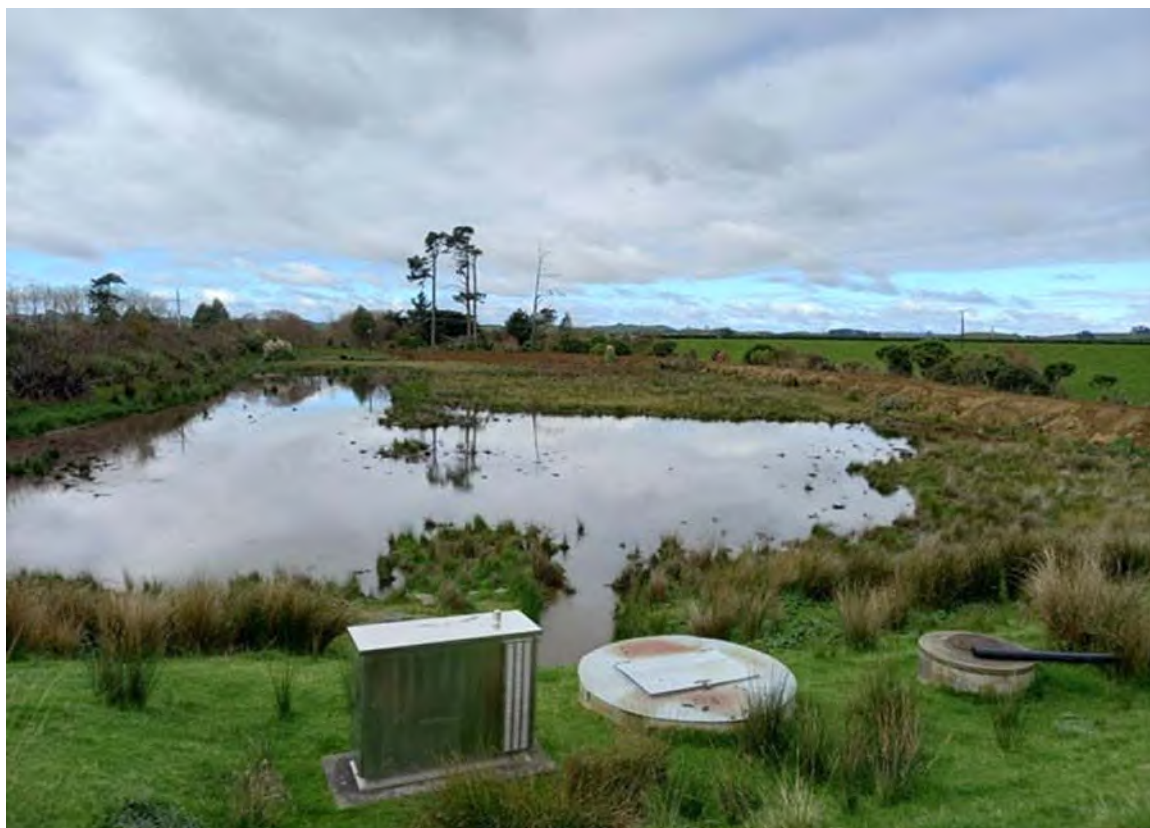
Photo 1 Overflow detention pond raised bund (right of photo)
