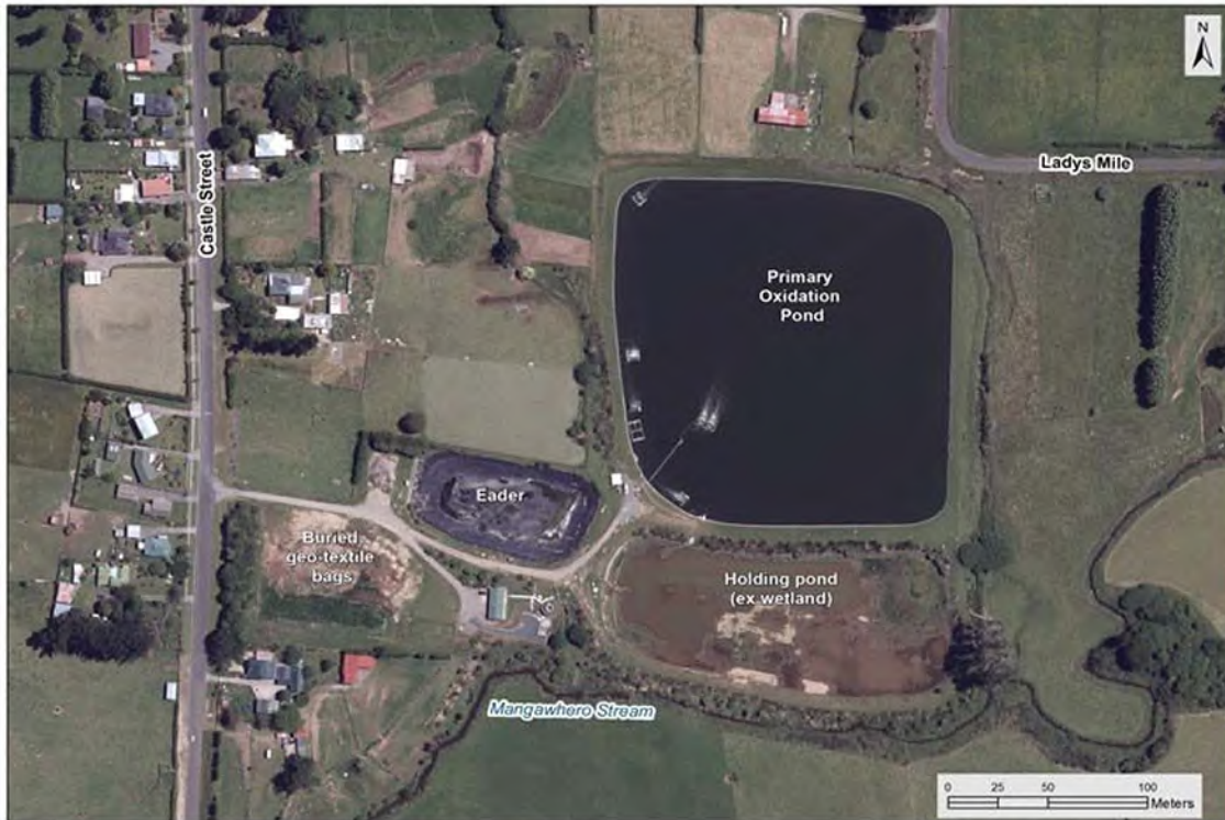
Figure 2 Aerial view of the Eltham WWTW
