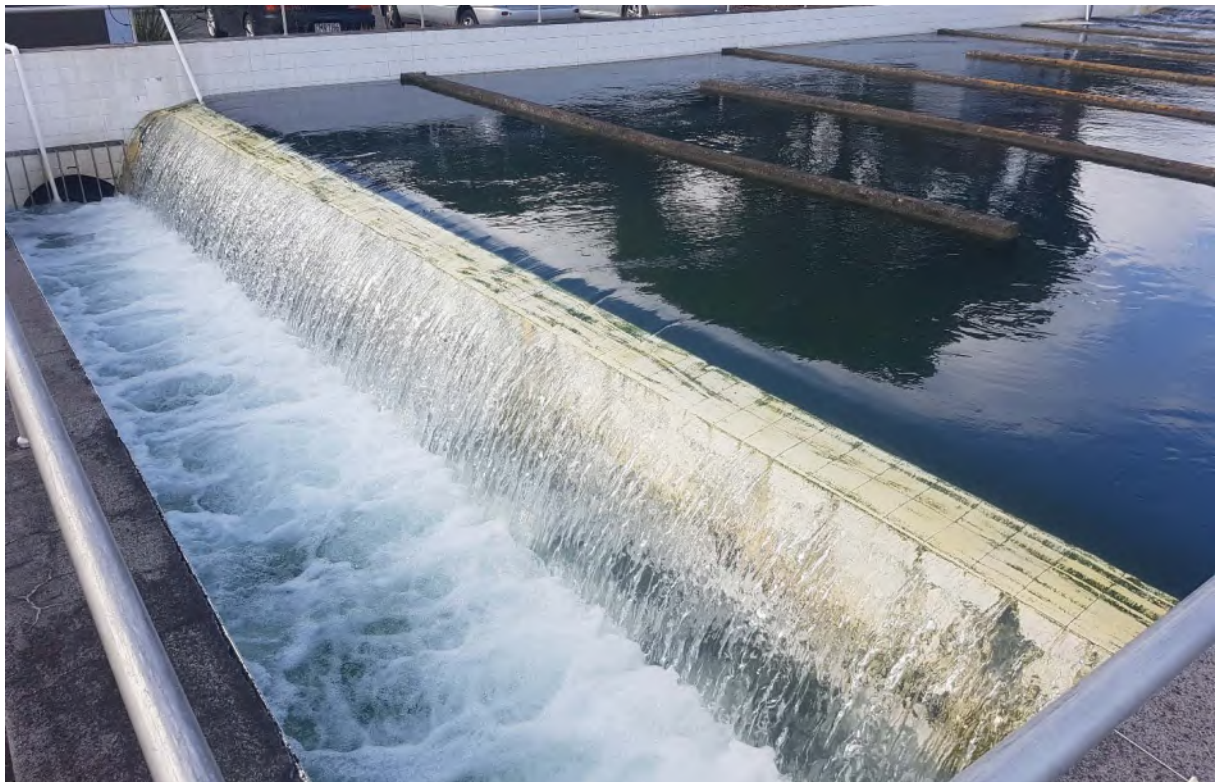
Photo 2 Final effluent discharging from the chlorine contact tank into marine outfall (11 December 2020)
