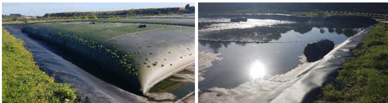
Photo 3 Geotextile dewatering bags (left) and dewatering filtrate draining back towards lagoon (right)
