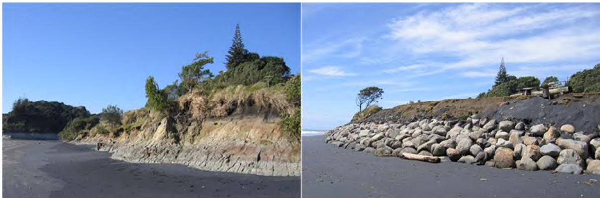
Photo 2 Erosion on Wai-iti foreshore prior to construction of the rock wall, and the rock wall facing north from stream (Nov 2005)
