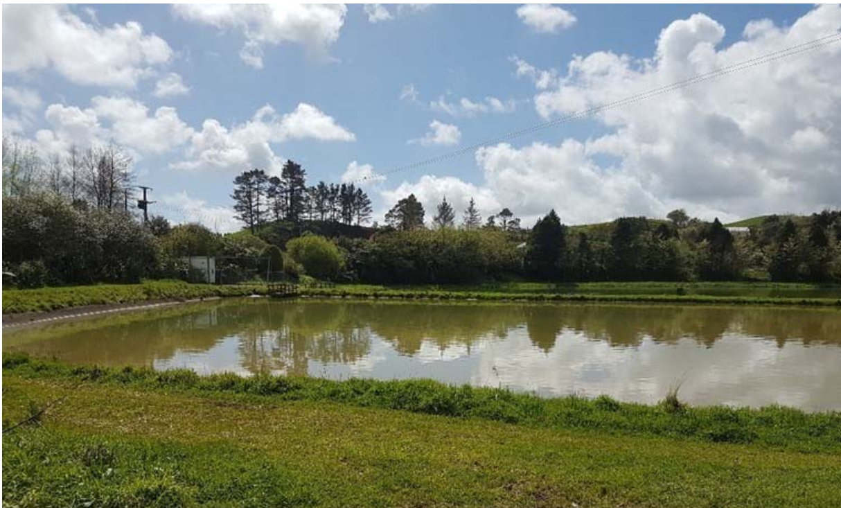
Photo 2 The Inglewood WWTP main pond
