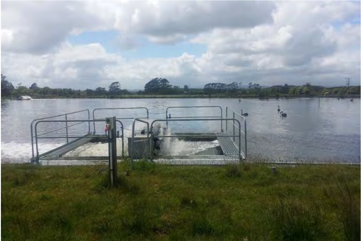
Photo 2 View of Stratford WWTP primary pond with aerators operating
