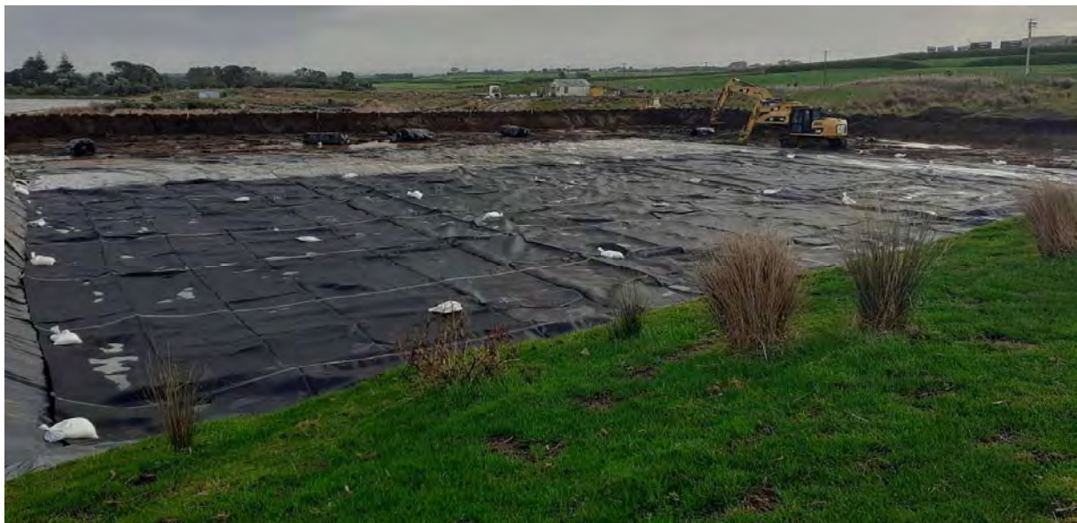
Photo 2 Nearly completed sludge dewatering area (July 2020)
