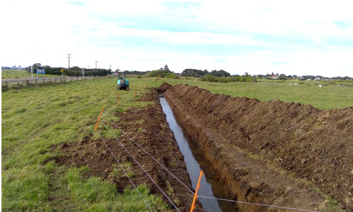
Photo 2 Excavation in the soakage field as part of an investigation into ponding
