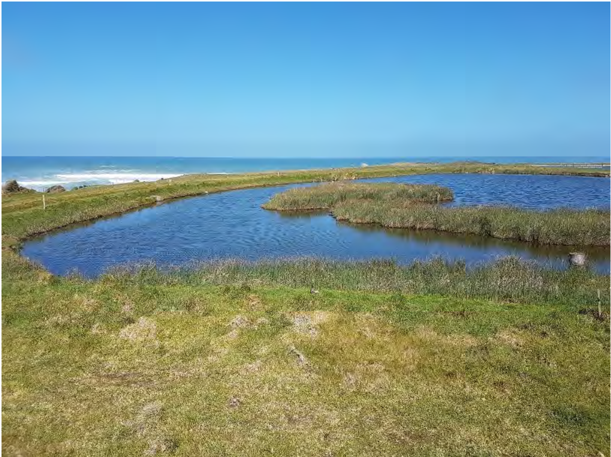
Photo 1 Opunake WWTP wetlands
