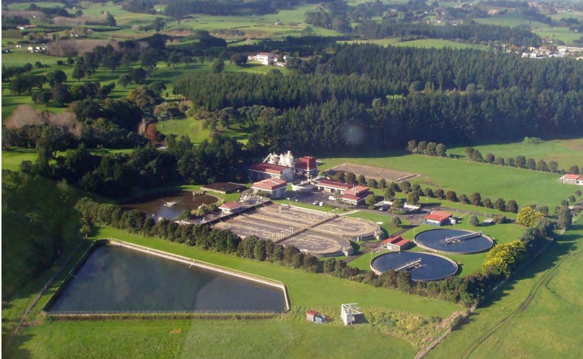
Photo 1 The New Plymouth Wastewater Treatment Plant
