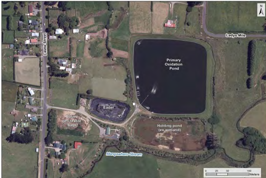
Figure 2 Aerial view of the Eltham WWTW
