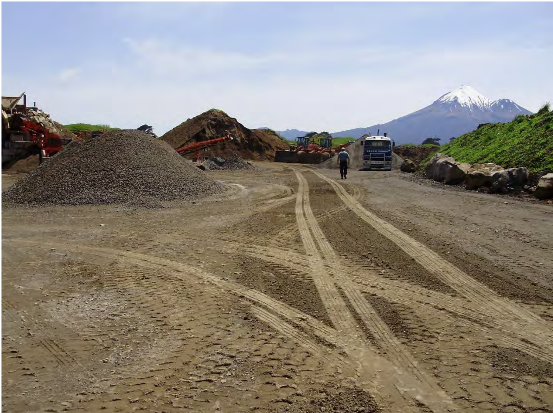
Photo 1 Waiteika Road quarry site 2009
