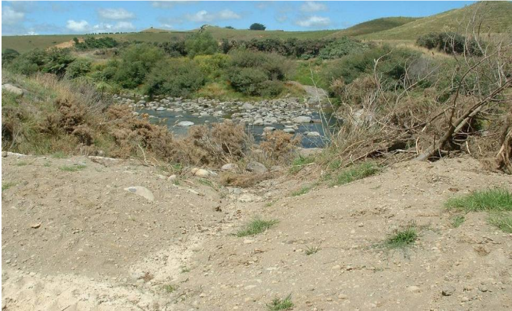
Photo 2 Stormwater discharge point to Waiwhakaiho River
