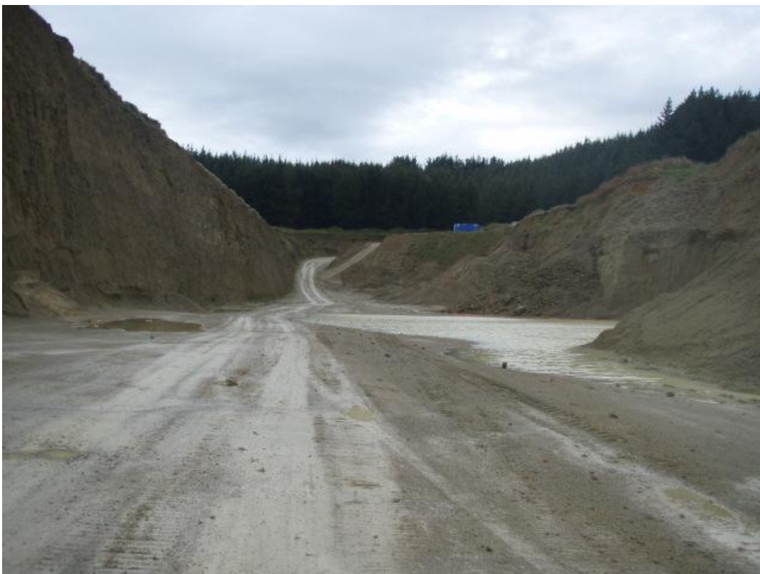
Photo 2 Stormwater collection area at base of quarry pit well away from Makokako Stream from which stormwater drains via seepage to ground
