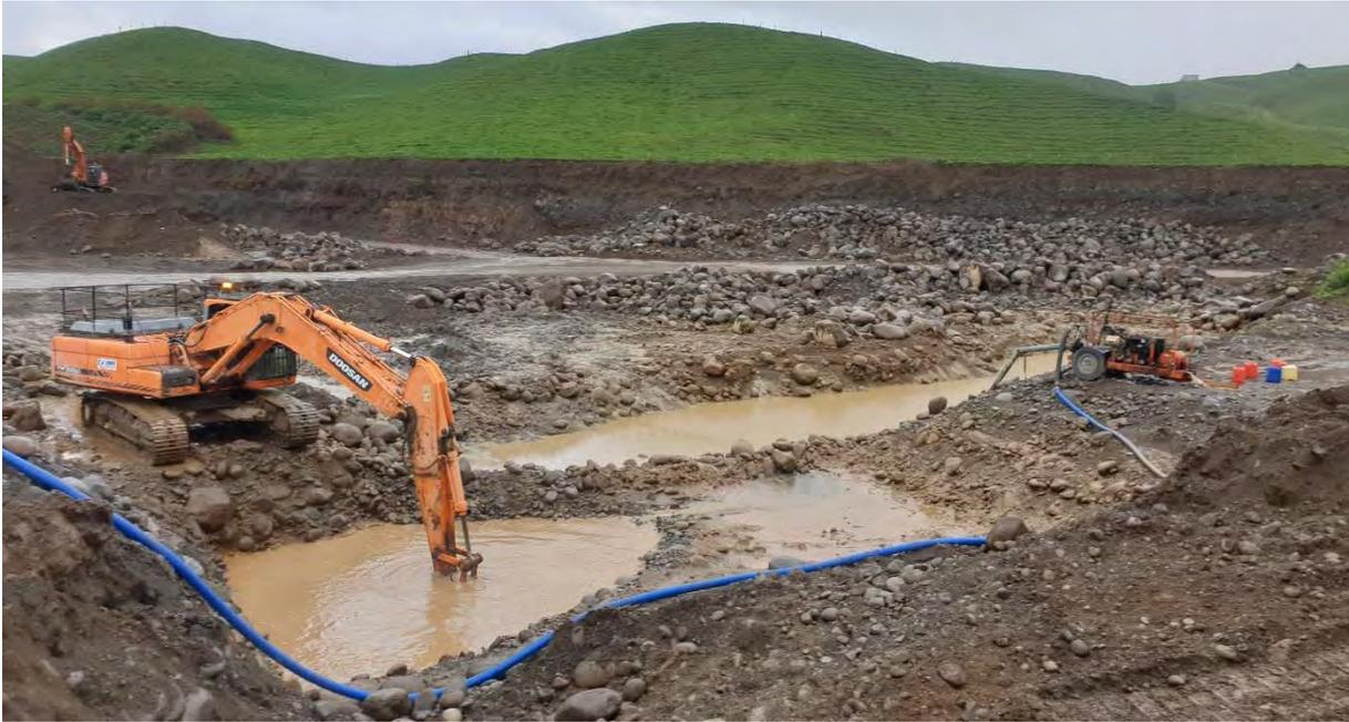
Photo 10 Hydro Road quarry construction of new settlement ponds, July 2019
