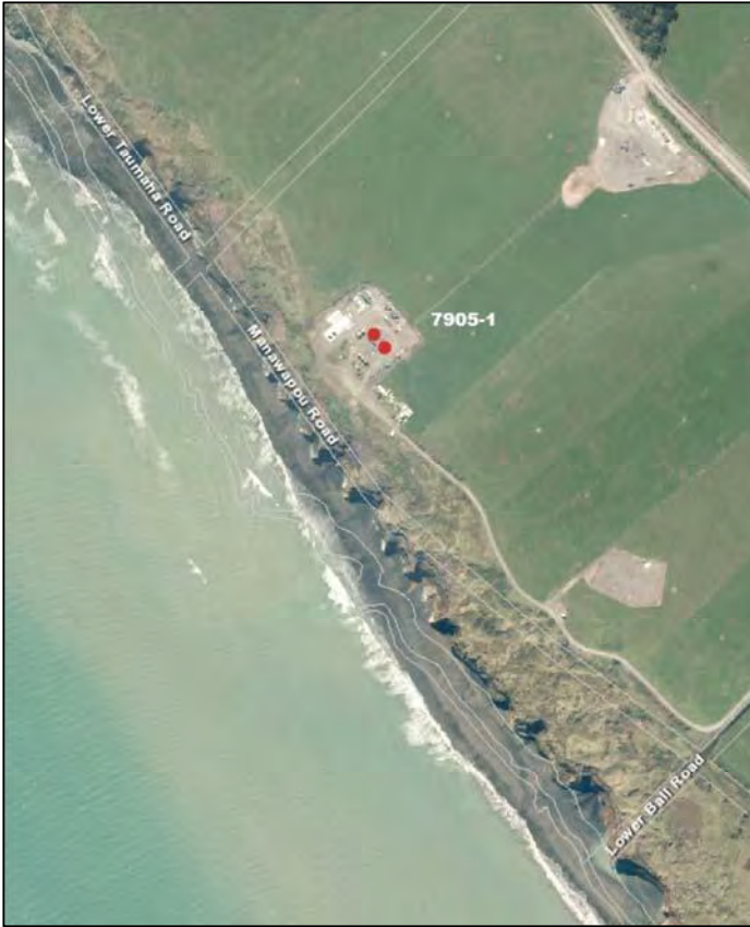
Photo 1 Manutahi-D wellsite and disposal wells D-2H and D-4H ST2 (7905-1)
