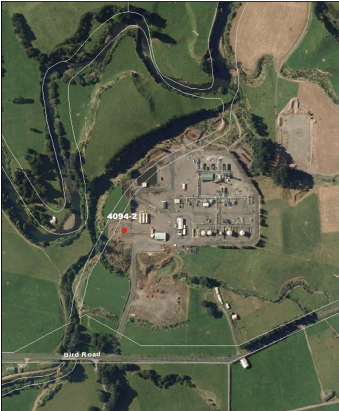
Photo 2 Waihapa-F wellsite and Waihapa-7A disposal well (4094-2)
