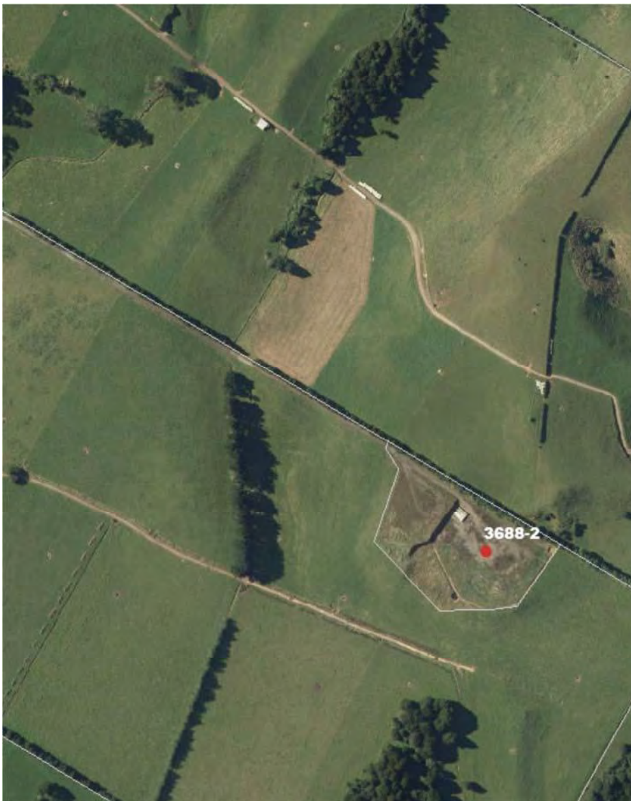
Photo 1 Waihapa-D wellsite and Waihapa-5 disposal wellsite (3688-2)
