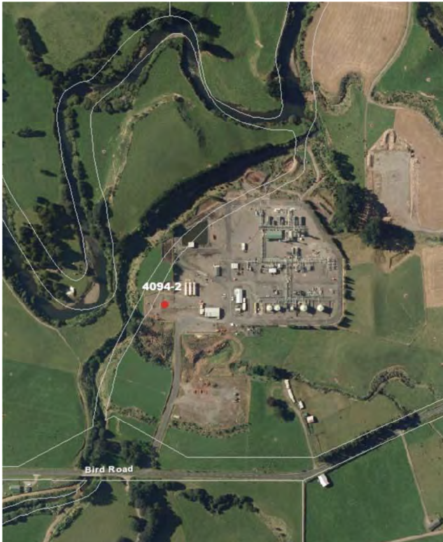
Photo 2 Waihapa-F wellsite and Waihapa-7A disposal well (4094-2)
